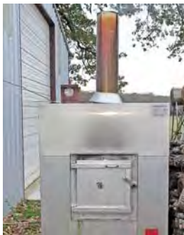
An outdoor wood-burning furnace provides most of the home's space-heating needs.
