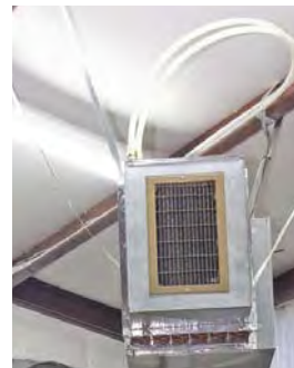
An open-loop heat exchanger provides warm air in the shop.
