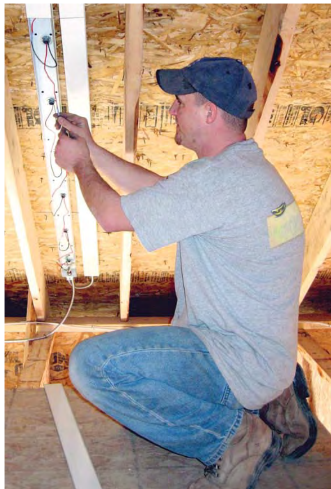
Making series connections in the raceway.
