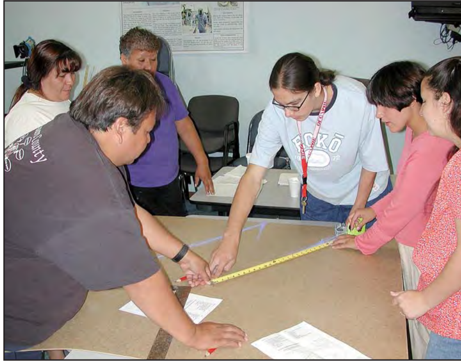
Laying out the pattern for a side reflector. After the measurements are transferred to the hardboard or plywood, use a chalk line to "snap" straight lines for the pattern pieces.
