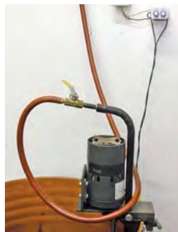
This drip oil-assist booster increases heat and reduces the amount of wood needed.
