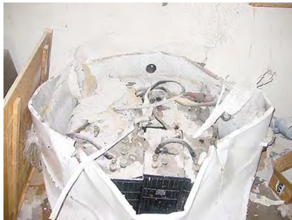
An extreme result of battery neglect.
