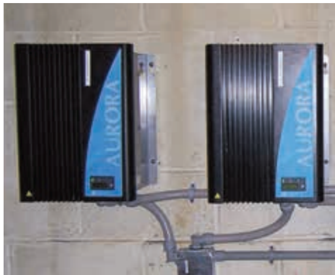
Two Power-One Aurora inverters synchronize the solar-electric system's output with the utility grid.
