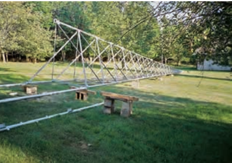
Assembling the top tower section.
