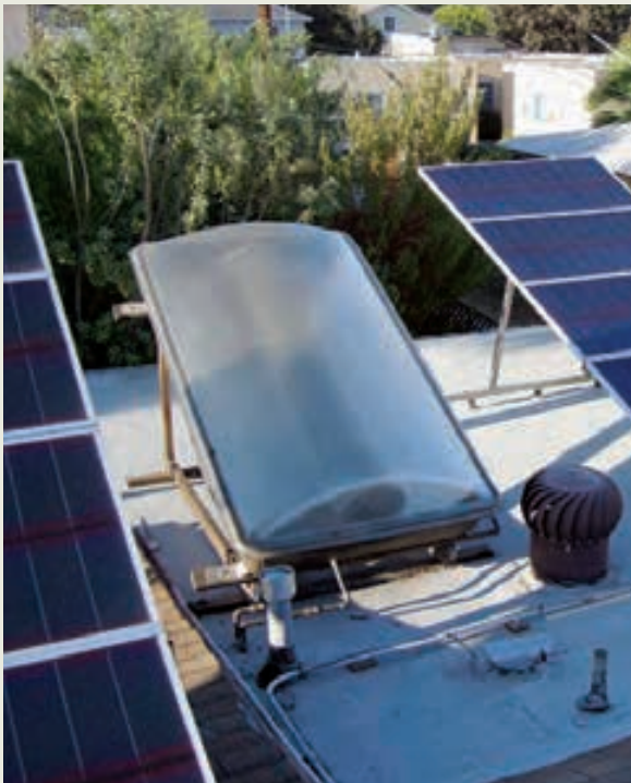
The Dolphins' solar batch heater reduces their water heating costs by half.
