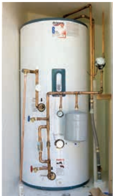
The almost-complete closed-loop plumbing. The original spring-type check valve was replaced.
