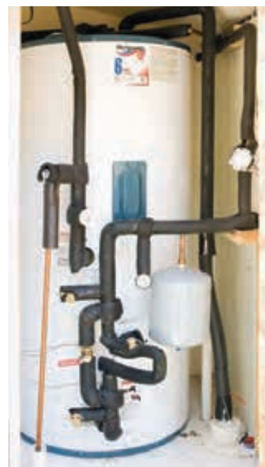
The completed plumbing, wrapped with high-temperature insulation and equipped with a swing-type check valve.
