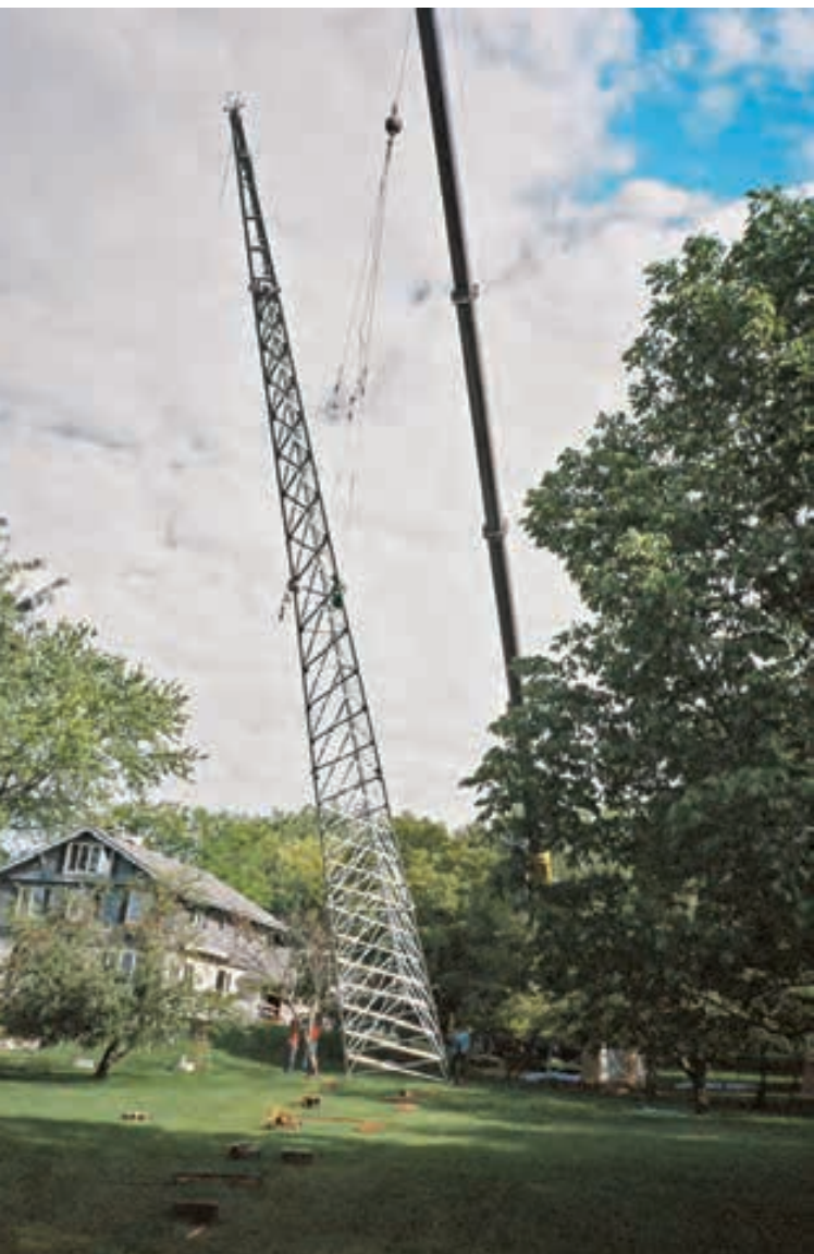
The crane lifts the 3,200-pound, 100-foot-tall tower section.
