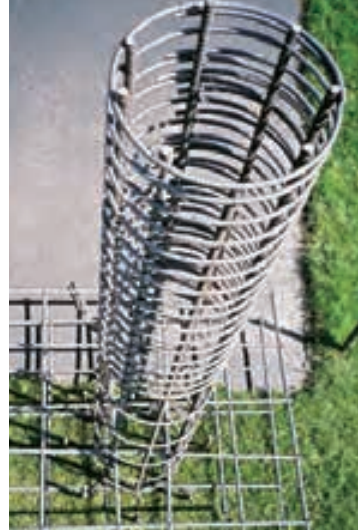
Prepping and pouring the footings for the tower. Far left: The excavated holes, with rebar cages in place. Center: Detail of rebar cages. Right: Tubular concrete forms are filled to form the upper 8 feet of the tower foundation.
