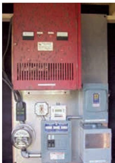
Left: The original Gemini synchronous inverter in its new home.
