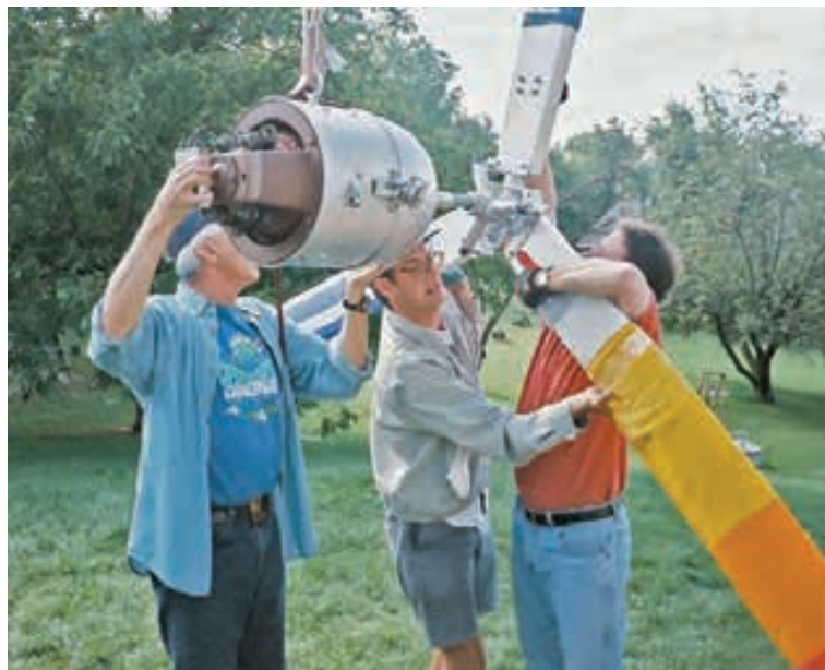
Mounting the rotor assembly to the generator. Temporary coverings protect the blades from damage.
