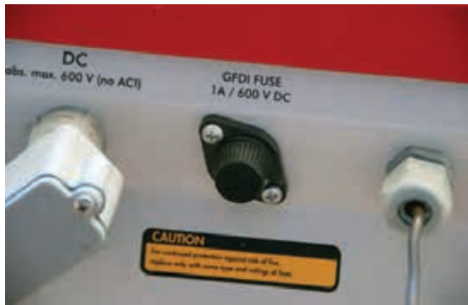
Ground-fault fuse location on a high-voltage inverter.
