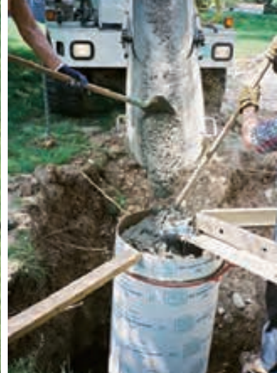
Prepping and pouring the footings for the tower. Far left: The excavated holes, with rebar cages in place. Center: Detail of rebar cages. Right: Tubular concrete forms are filled to form the upper 8 feet of the tower foundation.
