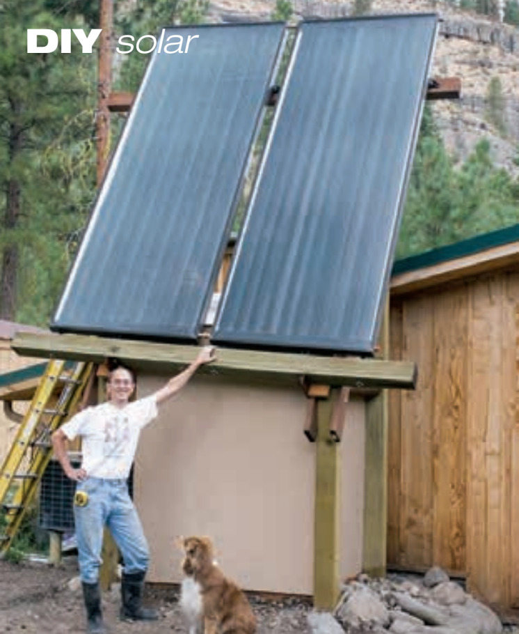
The flat-plate collectors in place, but not yet plumbed. The collectors were canted slightly to the right to facilitate drainage and thermosiphoning.
