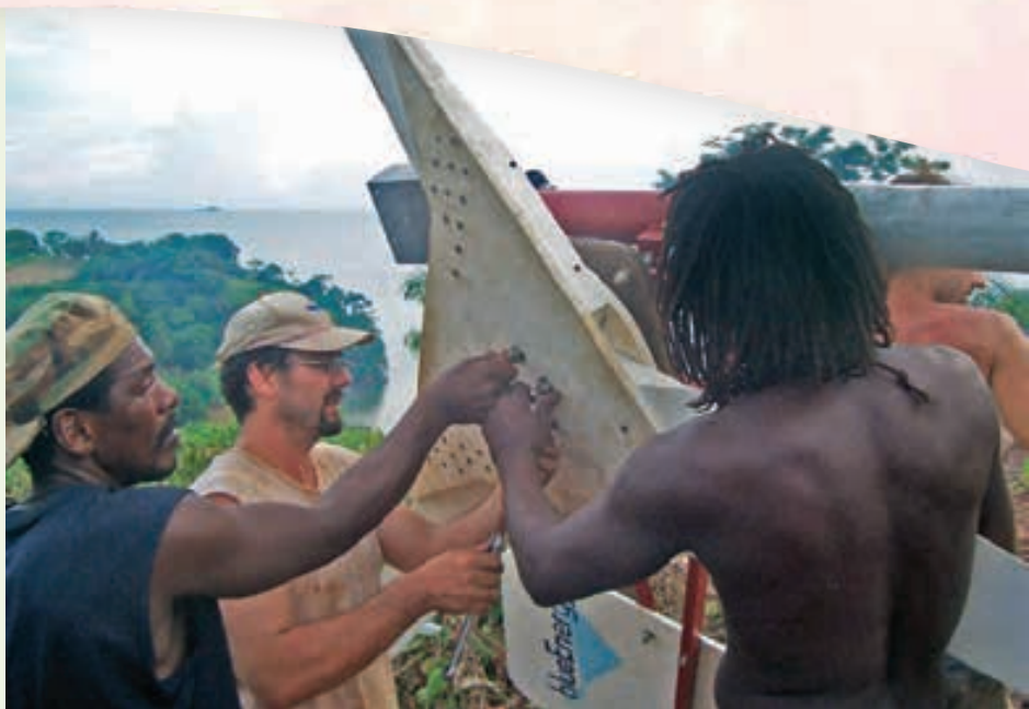
BlueEnergy’s Nicaragua director Guillaume Craig (center) works with community members to attach blades to the turbine.
