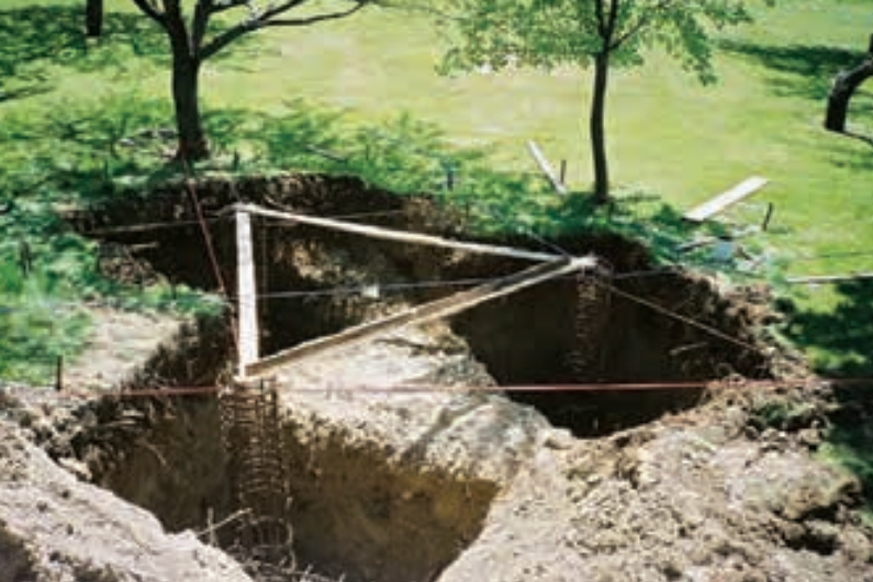
Prepping and pouring the footings for the tower. Far left: The excavated holes, with rebar cages in place. Center: Detail of rebar cages. Right: Tubular concrete forms are filled to form the upper 8 feet of the tower foundation.
