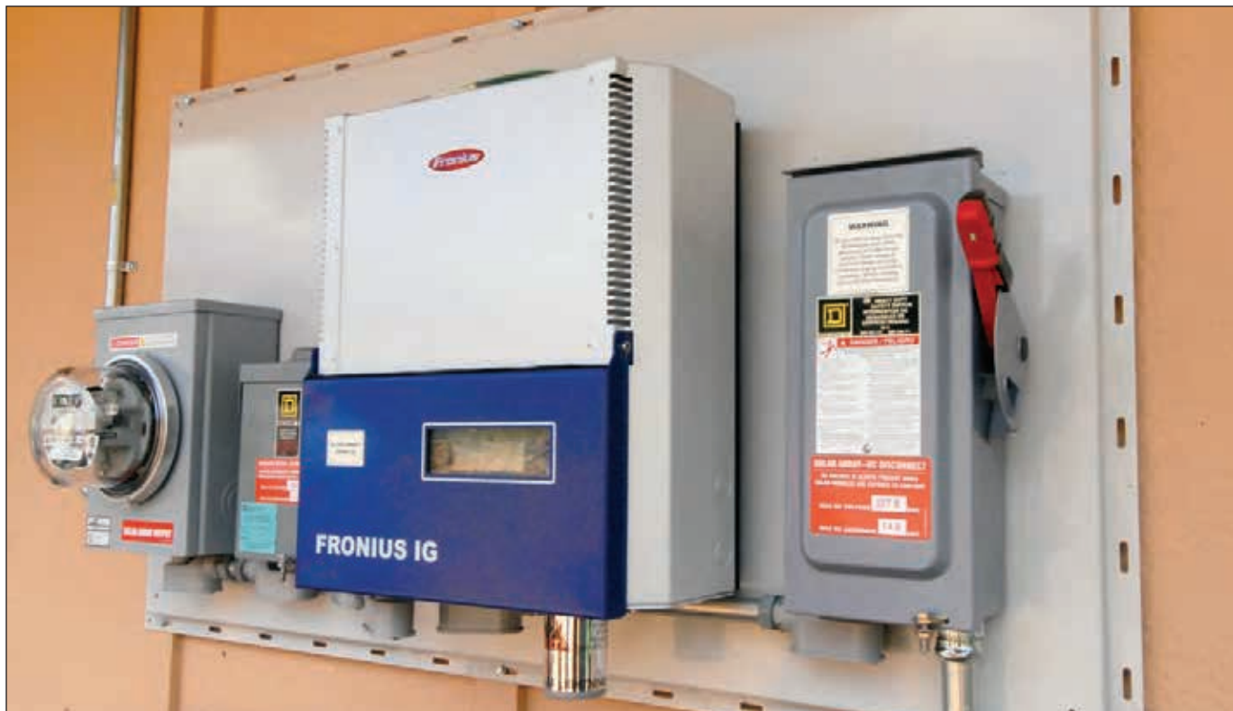
The power-conditioning and utility-feed components of a grid-direct PV system.
