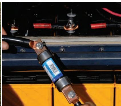
Assembling the interconnects and battery overcurrent protection. Far right: The neatly wired battery bank.
