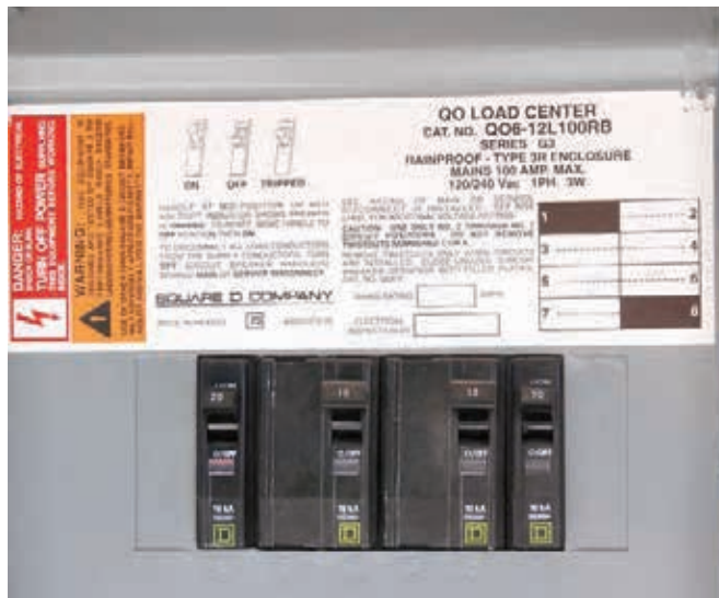
A main-lug-only panel, with no single main breaker. Use an empty breaker position for PV system input.
