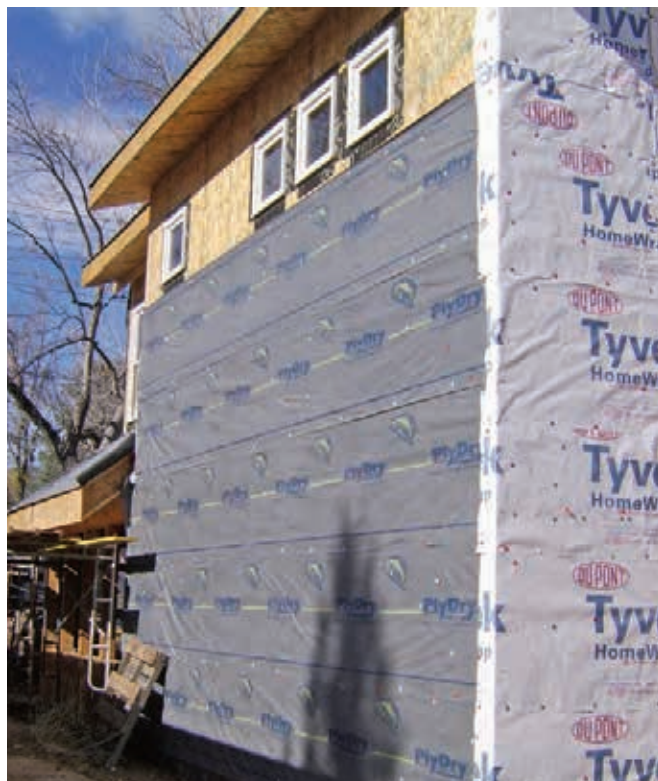
Properly installed house wrap acts as a barrier to the transmission of air and moisture.
