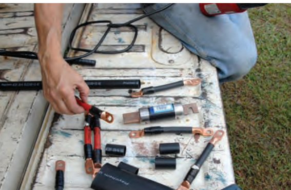
Assembling the interconnects and battery overcurrent protection. Far right: The neatly wired battery bank.
