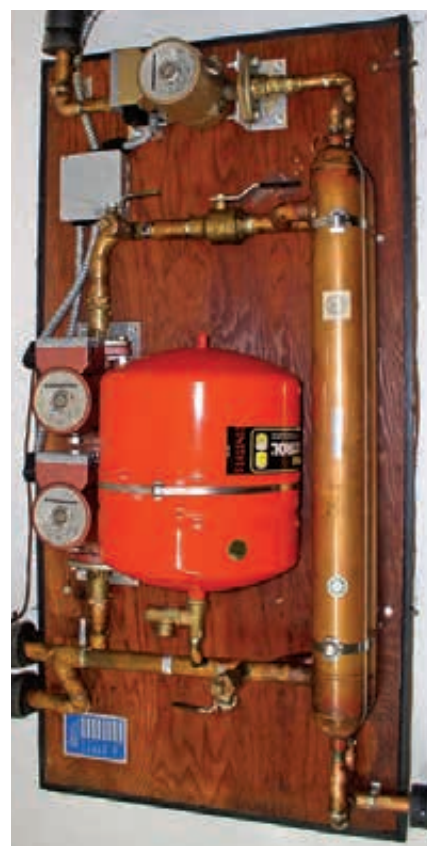
An external, tube-in-shell heat exchanger (far right) with other balance of system components, like circulator pumps (far left) and an expansion tank (center).
