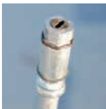
A cord grip keeps water, critters, and detritus out of a raceway, while allowing the cable to pass through.
