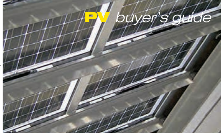
New technologies, like these Sanyo HIT modules, blur the divisions between traditional silicon types and gain higher efficiencies.
