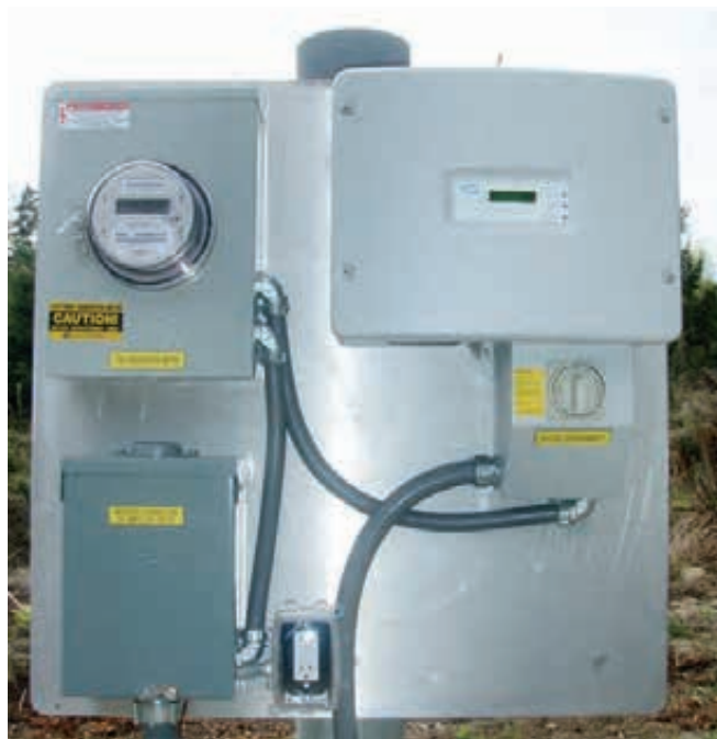
The simplicity of batteryless grid-tied balance-of-system equipment is hard to beat.
