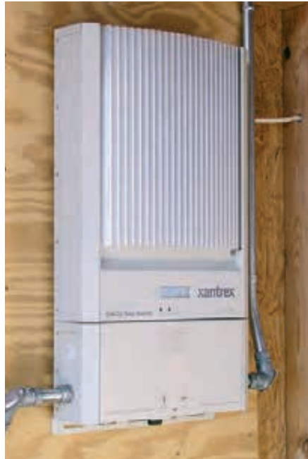
Left to right: The GridTek inverter for the wind system and the GT3.0 for the PV system.
