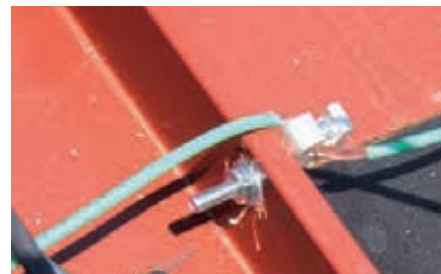
Oops: An indoor lug and wrong conductor type were used for grounding this standing-seam metal roof.
