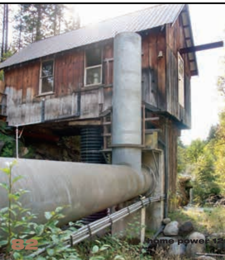
The penstock terminates at the powerhouse.
