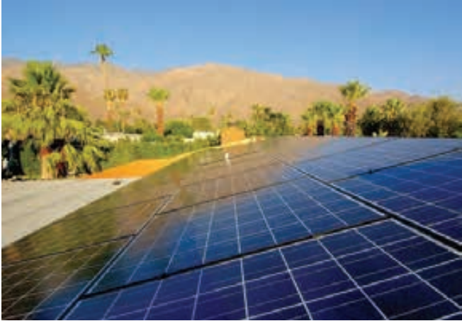
In lower latitudes, PV arrays with shallow tilt angles capture more of the sun's energy.
