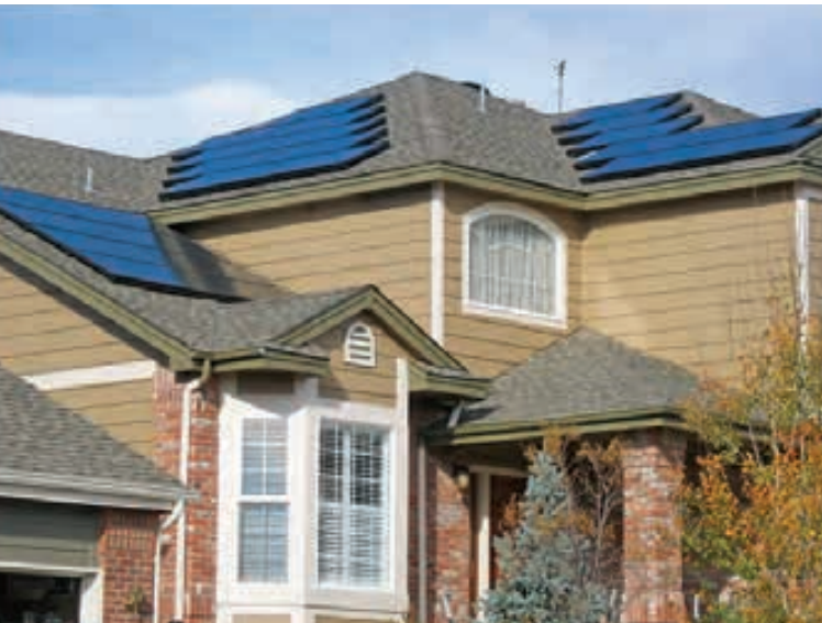
Subarrays at multiple orientations and tilts need special treatment, ideally independent MPPT inverters or charge controllers.
