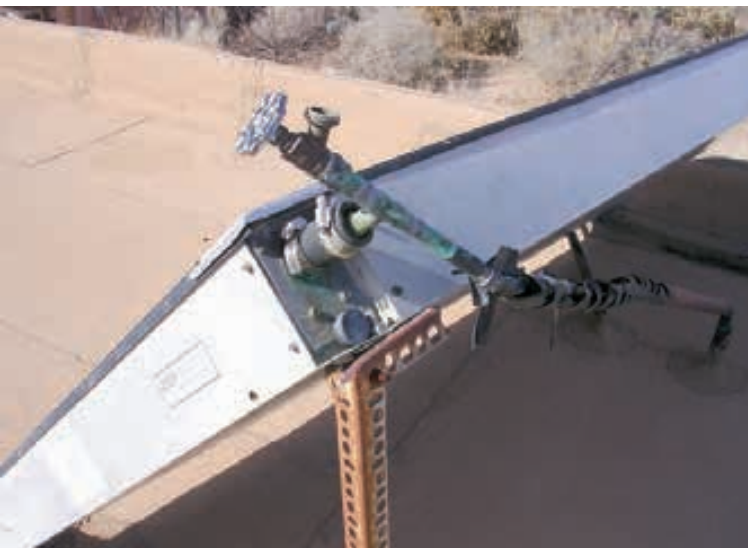
Although it's not pretty, this home-built mount-set has survived for more than two decades and still capably holds the collector.
