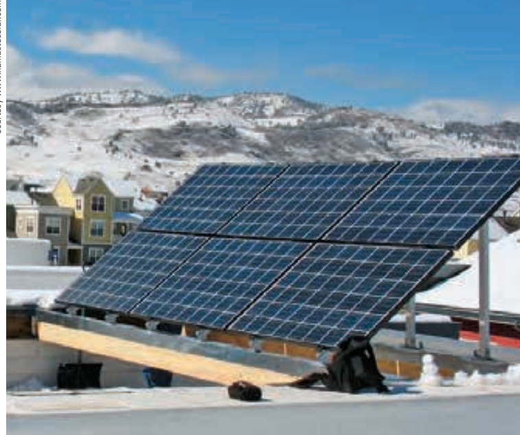
In higher latitudes, steeper tilt angles catch the low-angled sun and help the array shed snow more easily.
