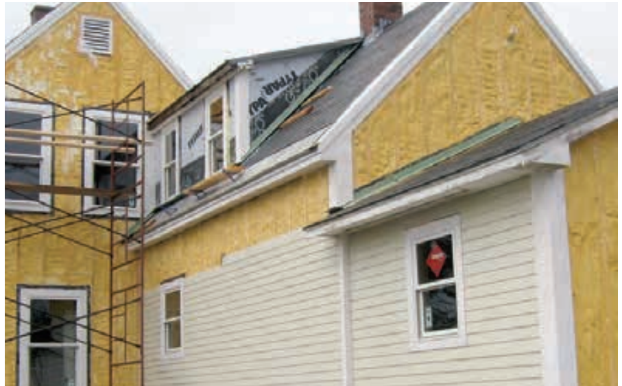
The asbestos siding was professionally removed, exposing another hazard underneath—lead paint-encrusted clapboard. A layer of closed-cell foam was sprayed over the old siding, encapsulating the paint and improving the home’s insulation.
