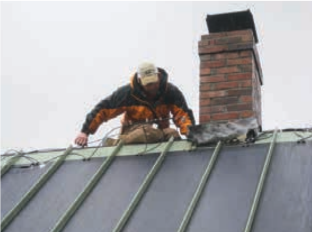
Clockwise from top: “Peel-and-stick” PV laminates are carefully applied on the new steel roofing pans. Installing the pans, just like any other steel roof. Modules are connected via wiring at the roof peak, which is covered with a ridge cap.
