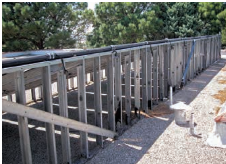
A pool heating system mounted on a site-built rack fabricated from steel studs.
