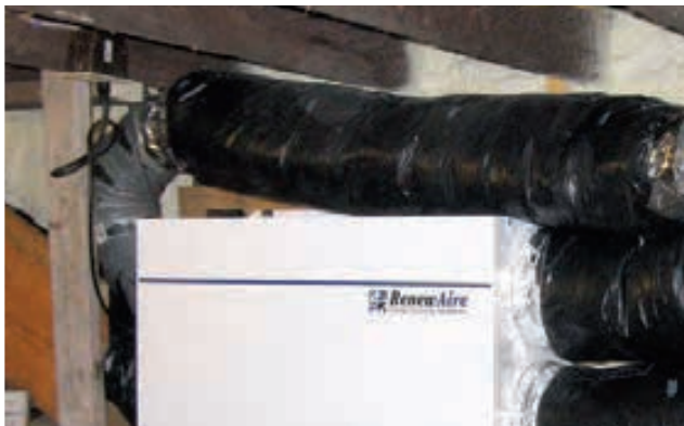
Above: The energy recovery ventilator brings fresh air into the home with minimal heat loss.
