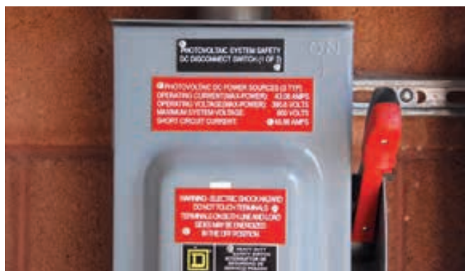
A properly labeled PV disconnect.
