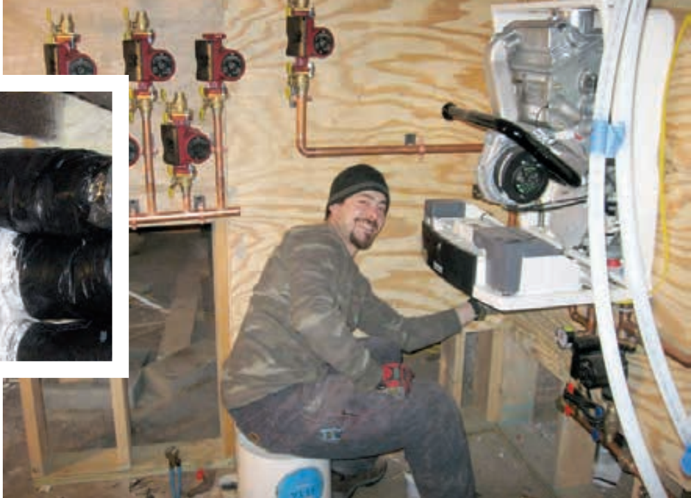
Right: The plumber installs the new boiler that will feed the new hydronic baseboard heaters.
