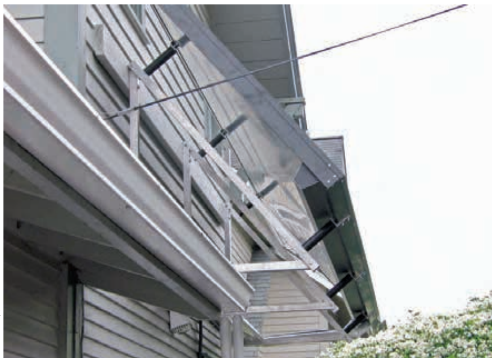
A wall-mounted collector with a mount-set that is long on function, but short on aesthetic appeal.
