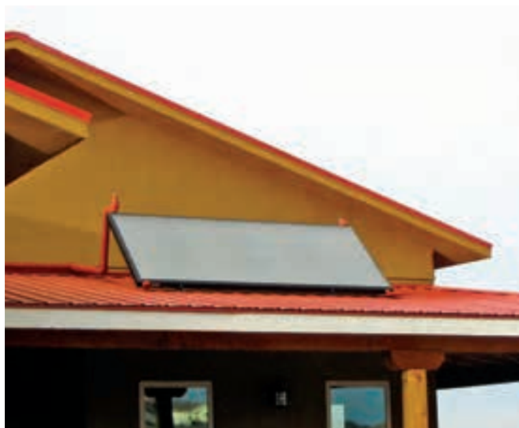
A flat-plate collector tilted to optimize winter performance.
