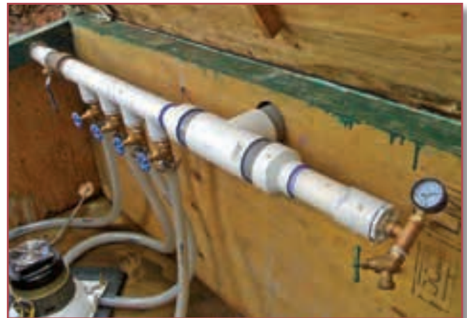
Four valves control flow to the four nozzles, while a pressure gauge monitors system head.
