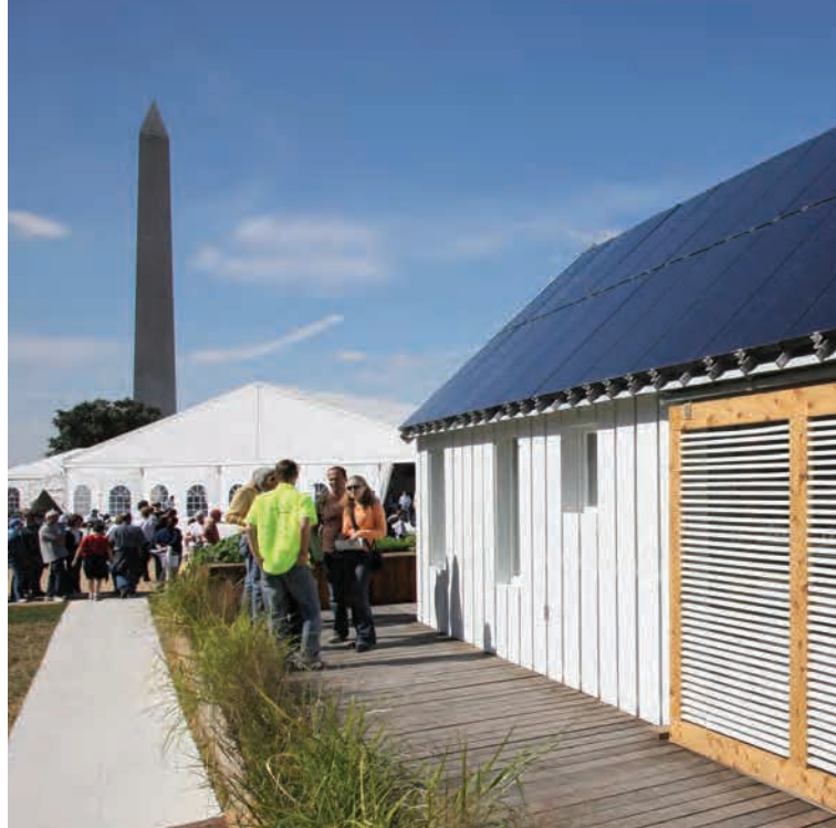
Beneath its recycled barn-wood cladding, the University of Illinois' Gable Home features super-insulated walls and ceilings.
