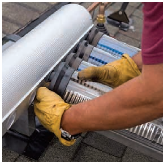
Inserting the evacuated tubes into the header.
