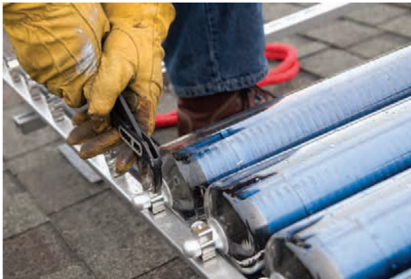
Clipping the bottom of the tubes into the lower end of the rack.
