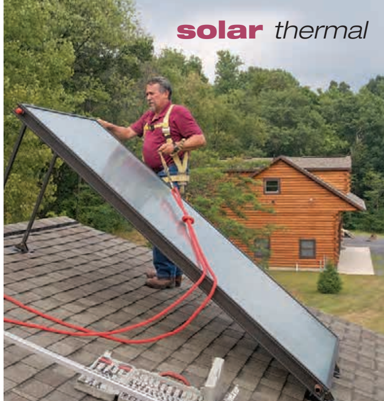
The Oventrop flat-plate collector is installed on the house's roof (the detached garage is in the background).
