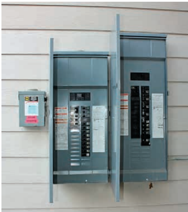
The PV system disconnect (left) next to the AC service entrance (middle) and the subpanel for loads backed up by the battery-based system (right).
