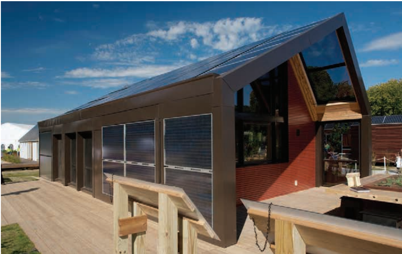
Conventional BP and Sanyo bifacial PV modules are integrated into the roof and façade of the University of Minnesota's ICON Solar House.
