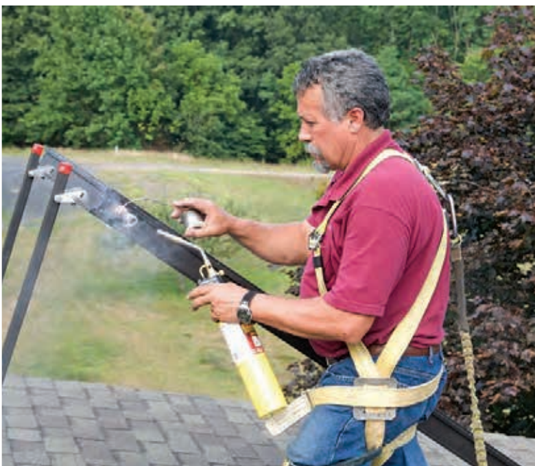
The sweating of the thermal line-sets begins.
