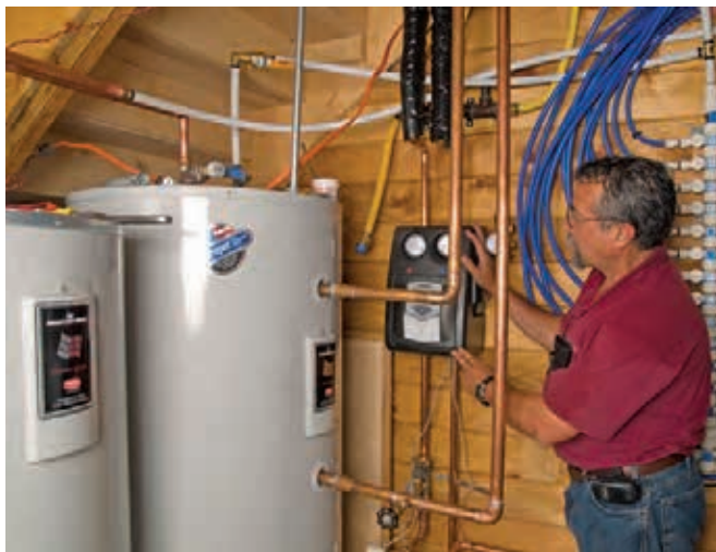
Storage tanks and pump-stack/controller.
