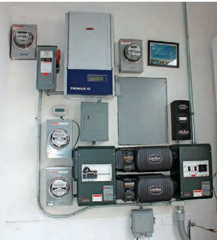
Grid-direct and battery-based PV systems share the same wall space. While three of the meters shown are PV production meters, the meter at the upper left is simply to measure kWh consumption of the electric space heaters.
