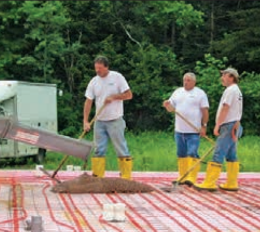
Step 6: Pouring and distributing the concrete.
