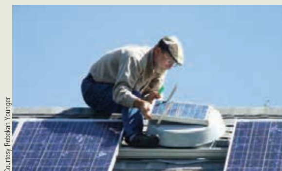
Adjusting the small PV module on the attic fan helped reduce shading on an adjacent module.
