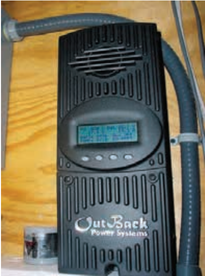
Step-down MPPT controllers can help decrease wiring costs by allowing PV array voltage to be higher than the battery bank voltage.
