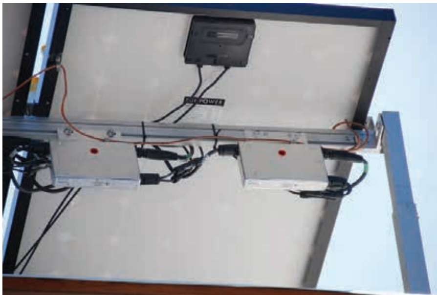
Two Enphase inverters, showing their DC input connections, and AC input and output connections.
