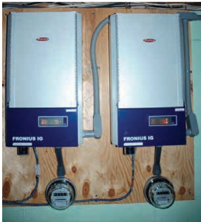
Two Fronius grid-tied inverters make up the balance of the home's photovoltaic system.
