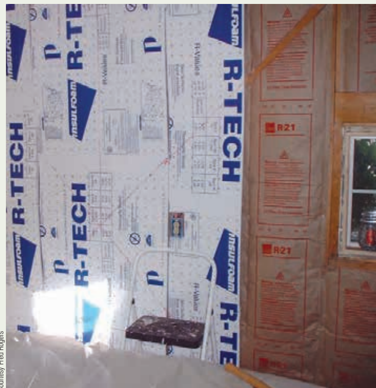
Insulation upgrades included rigid foam-board (at left) over R-21 fiberglass batts (on right).
