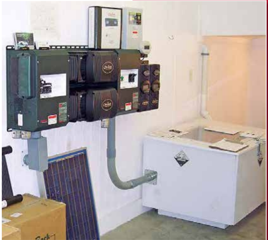
Above: Two stacked inverters are the core of this OutBack system, which integrates charge controllers and other BOS components.
