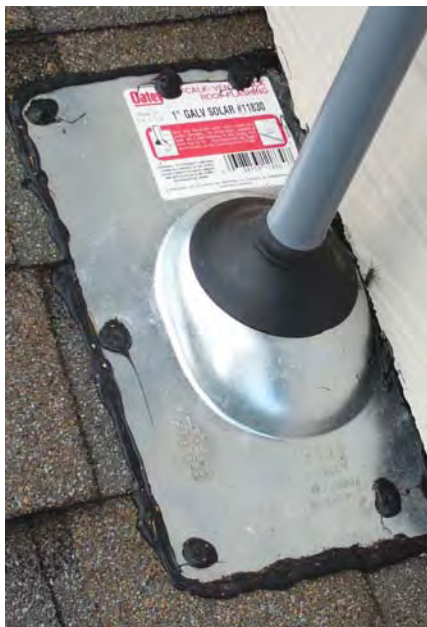
Unlike the example shown at left, roof penetrations need to be properly flashed. Always follow the equipment manufacturer's instructions during installation.
