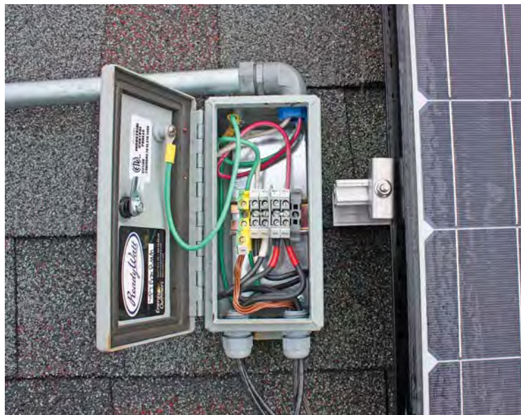
A transition box can be used to change wire types and sizes on the roof.
