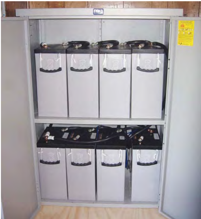
This battery enclosure allows for stacking batteries, reducing the footprint required. This is one clear benefit of sealed batteries, as access to cell caps to add water is unnecessary.
