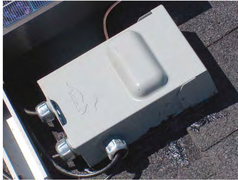
NEMA 3R-rated boxes should not be installed at angles less than 14 degrees.
