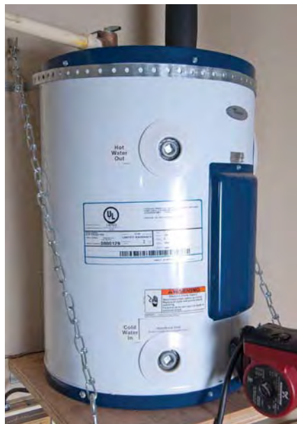
Above: A small electric water heater is used as a drainback tank, allowing heat-transfer fluid to drain from the collector when the system is not operating.
