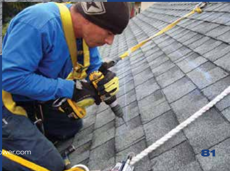
Right: Drilling a pilot hole to verify rafter position. If the drill punches through after going in less than an inch, you didn't hit a rafter. Size your pilot hole to match the necessary hole size for your lag bolts ( \frac{1}{8} in. is common).
