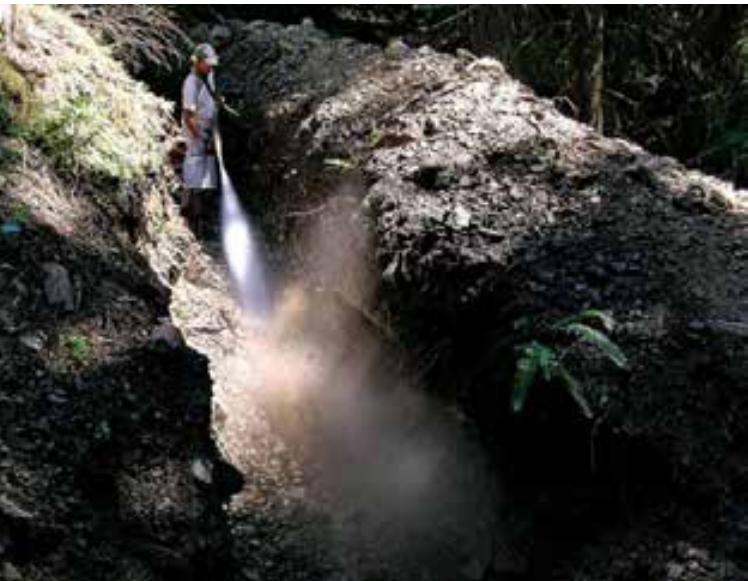
Water pressure was used to blast the trench for the lower penstock.
