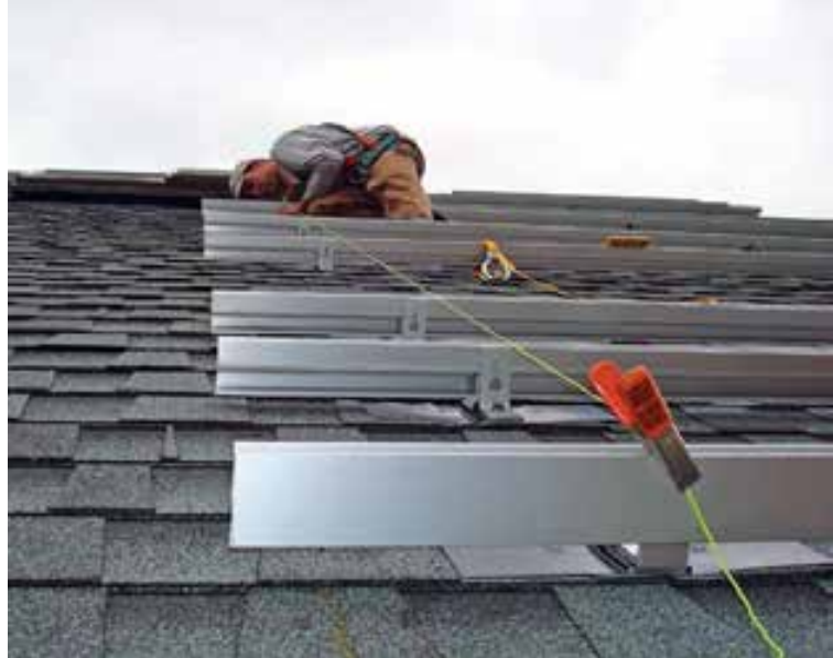
Leveling mounting rails with a string line.
