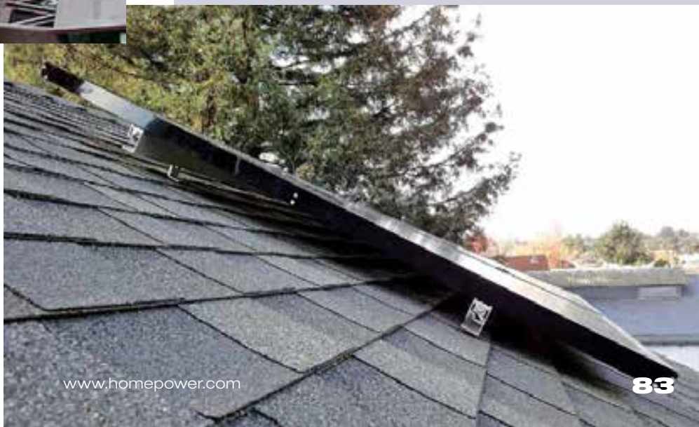
Above: Sighting along the edge is often enough to align PV modules accurately.
