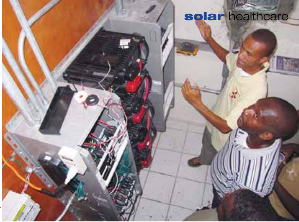
Students review the wiring of the OutBack Power system.
