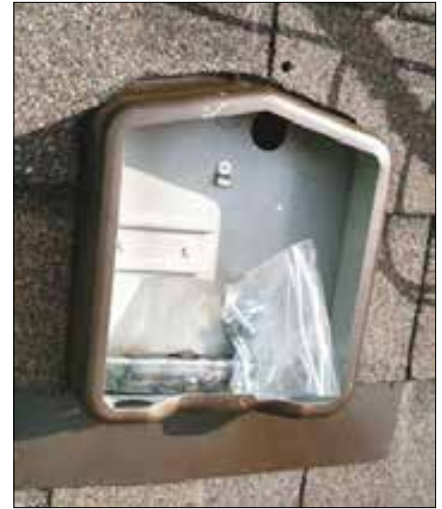
The SolaDeck junction box was painted to match the roof.
