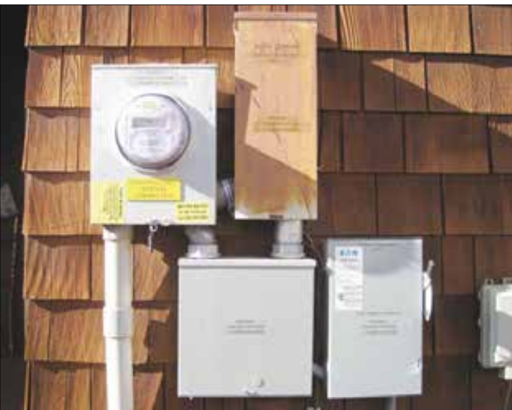
The AC side of the system with supply-side connection. The PV AC fused disconnect is at the bottom right. The junction box (bottom left) splices the output of the PV AC disconnect to the utility lines from the meter (upper left) and to the main service disconnect (above disconnect and junction box).
