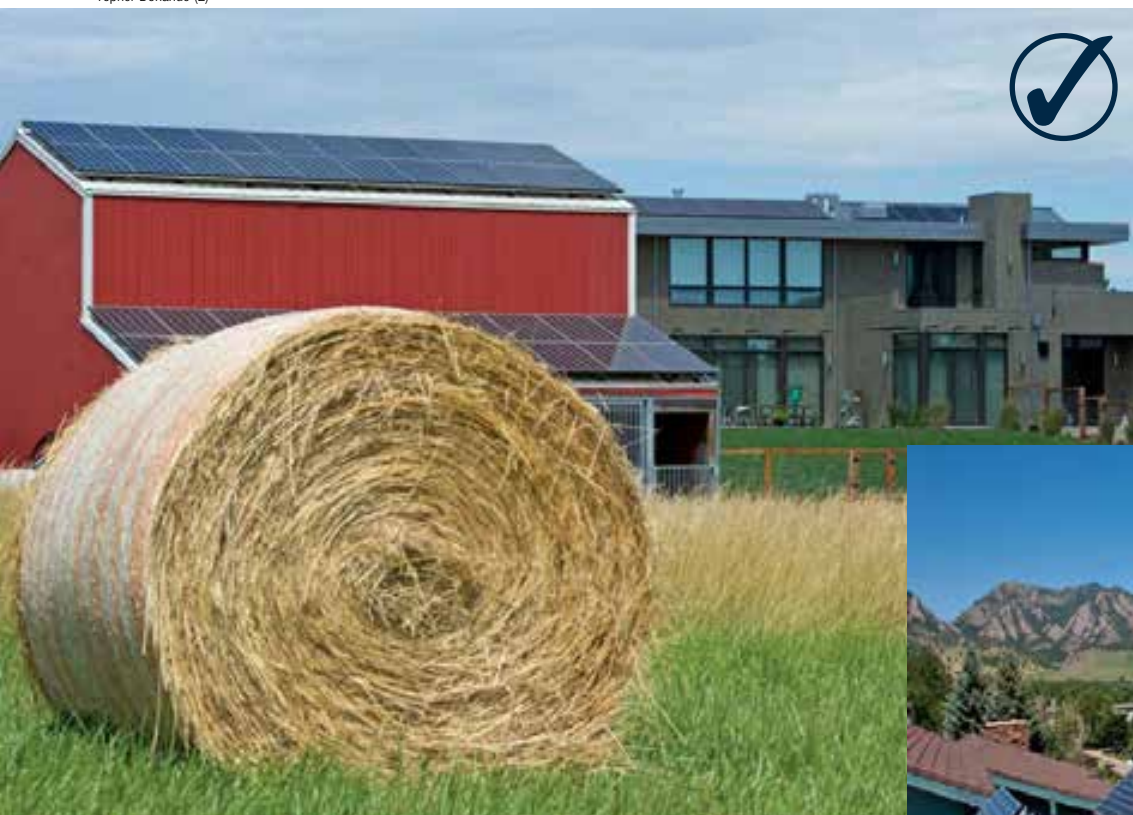
Above: Even on very low-angled roofs, PV arrays mounted parallel to the roof plane can produce a significant percentage of their potential, with a streamlined appearance.
