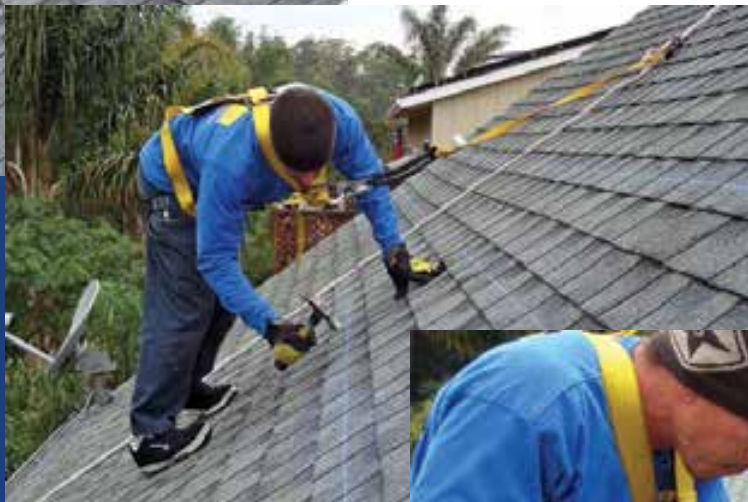
Right: Drilling a pilot hole to verify rafter position. If the drill punches through after going in less than an inch, you didn't hit a rafter. Size your pilot hole to match the necessary hole size for your lag bolts ( \frac{1}{8} in. is common).
