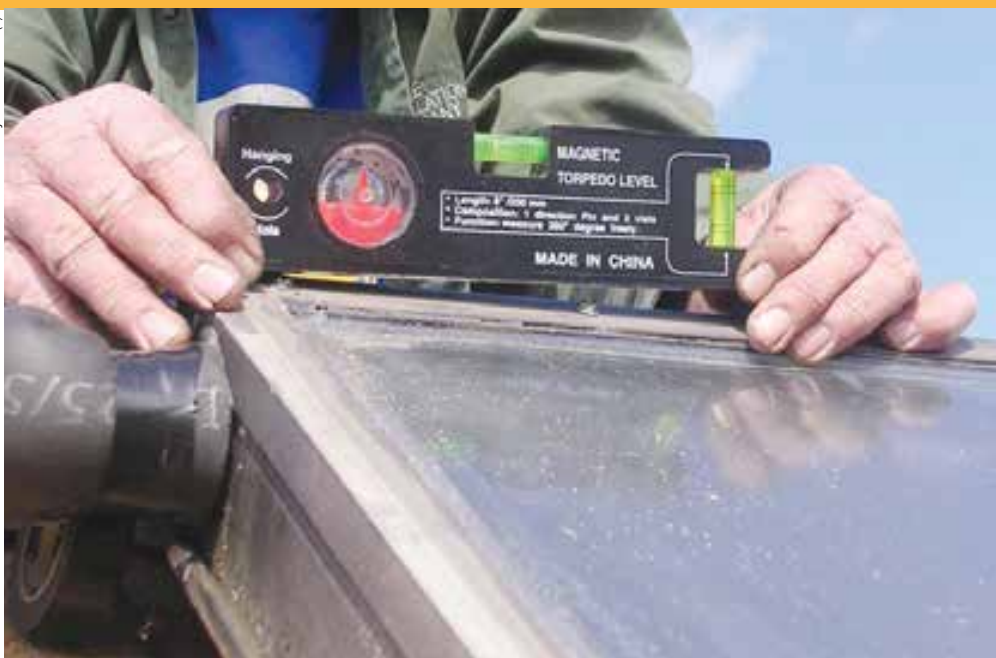
All plumbing, including the collectors, in a drainback system is sloped to allow the system to drain.
