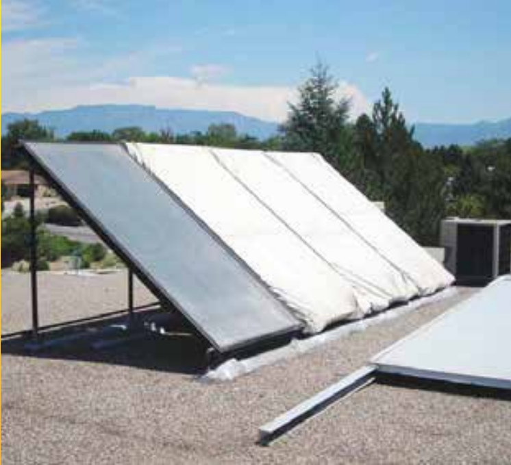
Covering some of the collectors will provide protection from summertime overheating.
