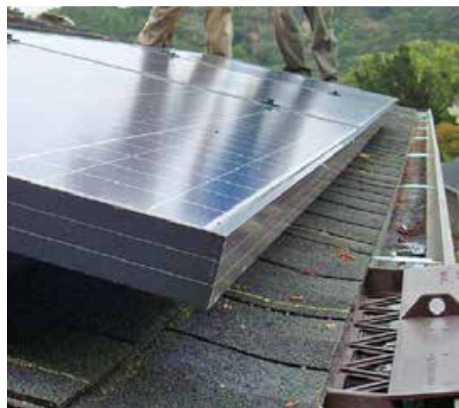
Above: Sighting along the edge is often enough to align PV modules accurately.
