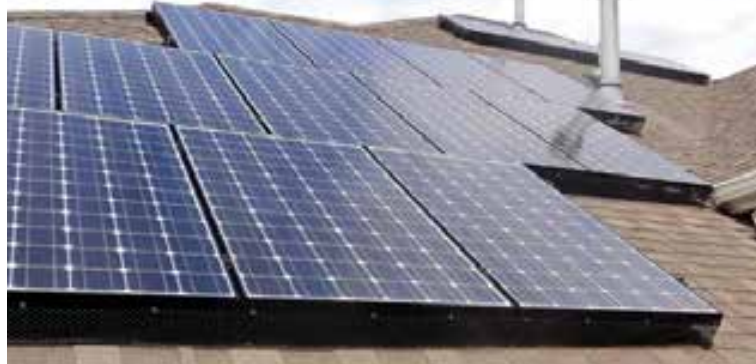
Complex roof angles, obstructions, and shading all affect options for array position. (Note the screen under the array to keep out varmints.)
