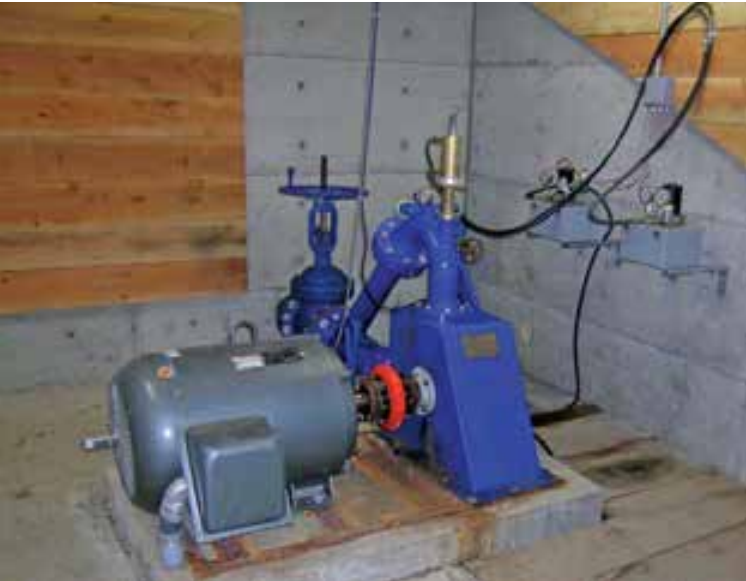
The Canyon Industries turbine consists of a 10.5-inch Pelton turbine and a 60 kW, 480 VAC, three-phase alternator.
