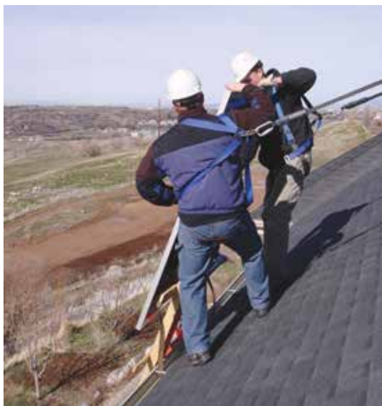
The secured module is hoisted from the ground to the crew on the roof.
