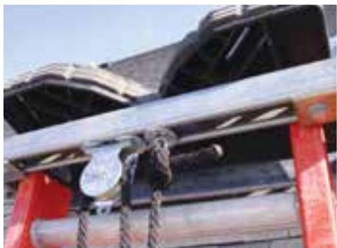
The author places the pulley support on top of the ladder.
