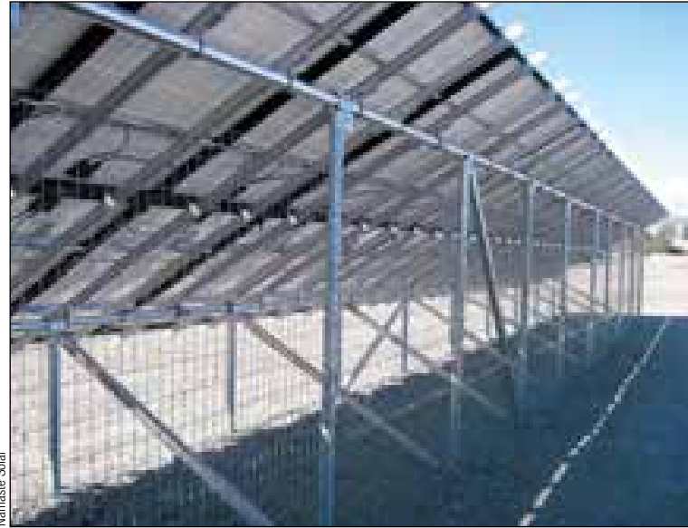
Fencing may be required, and may prevent animals—including the human kind—from tampering with array wiring.
