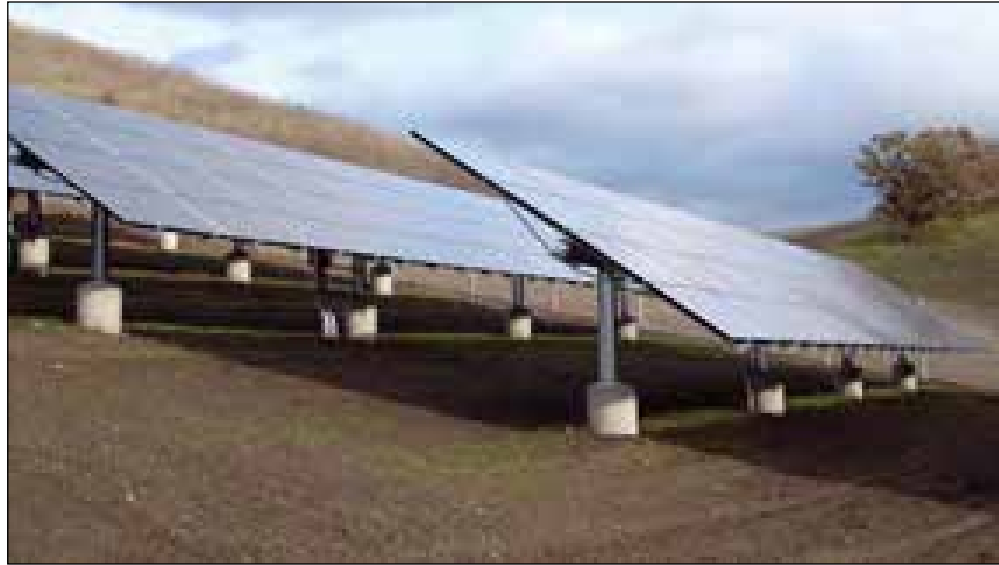
Arrays on single-row multipole ground mounts can be adjusted seasonally to optimize production. Arrays must be spaced carefully to avoid shading each other.
