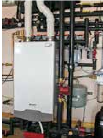
A Triangle Tube propane boiler makes up for what the solar collectors don't supply.
