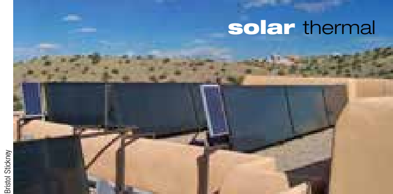
Solar thermal collectors provide the majority of domestic hot water and space heating for this Southwestern home.
