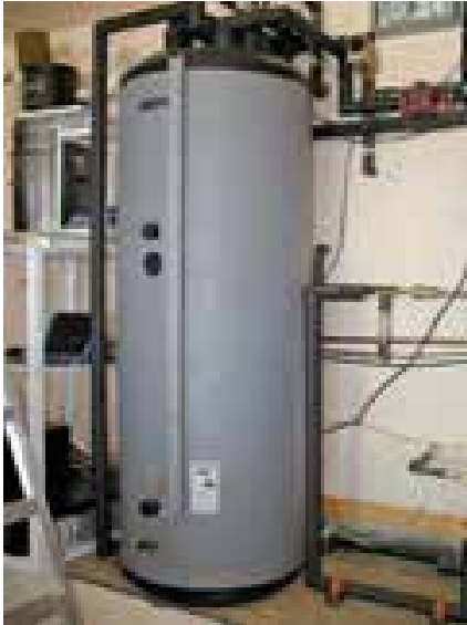
The domestic hot water tank does not have a heat source, but heats through internal exchangers from the primary loop and directly from the backup boiler.
