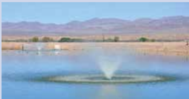
PV-direct water or air pumps can provide aeration and/or freeze protection.
