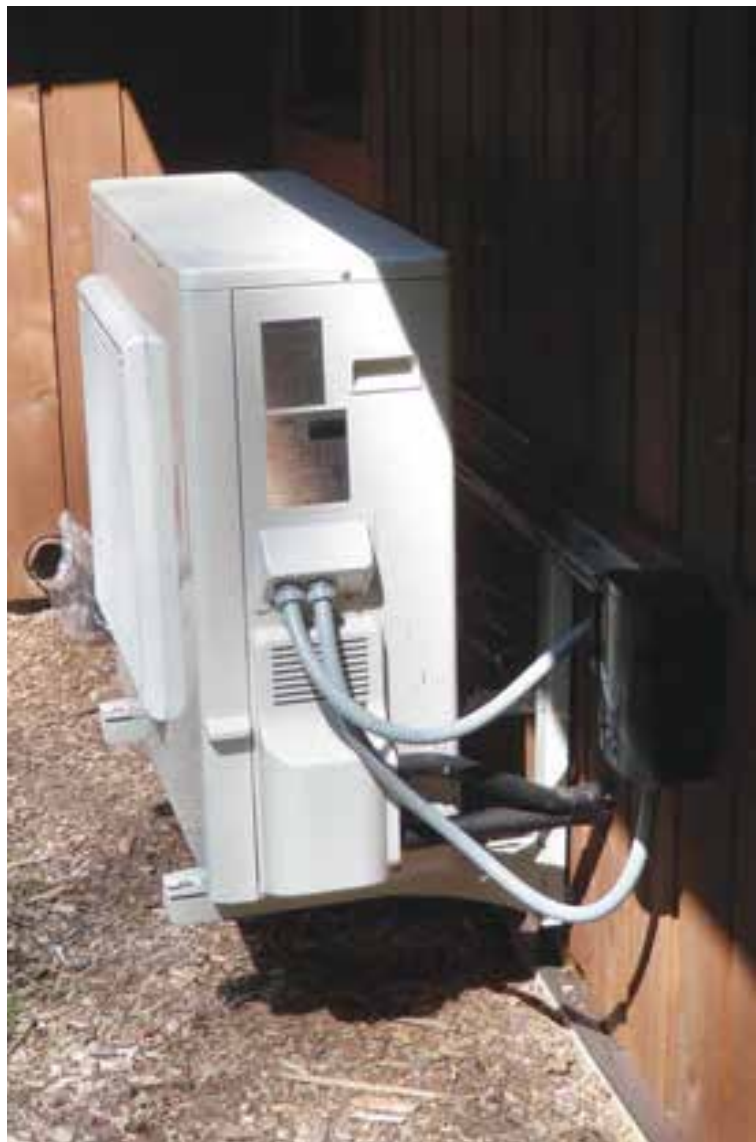
The outdoor unit of a mini-split air conditioner and heat pump.
