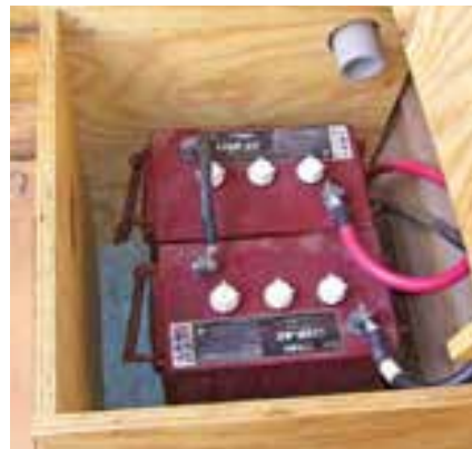
Two Trojan L16E-AC batteries provide 370 Ah of energy storage.
