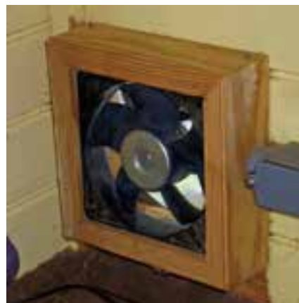
Right: The DC circulation fan draws cool room air into the bottom of the collector. Powered PV-direct, the air flow is proportional to the amount of sun.
