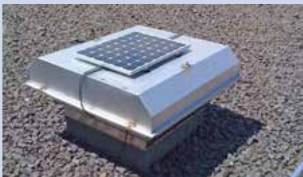
The stronger the sun shines, the more air this PV-direct ventilation fan exhausts.
