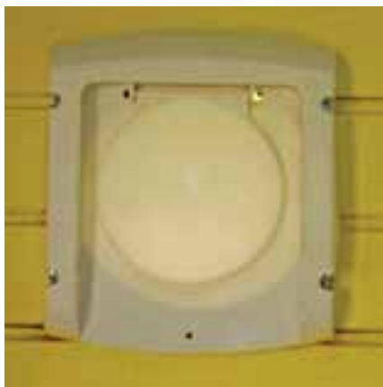
Left: A backdraft damper vents warm air into the office space from the top of the collector, but prevents reverse convection at night or during cloudy weather.
