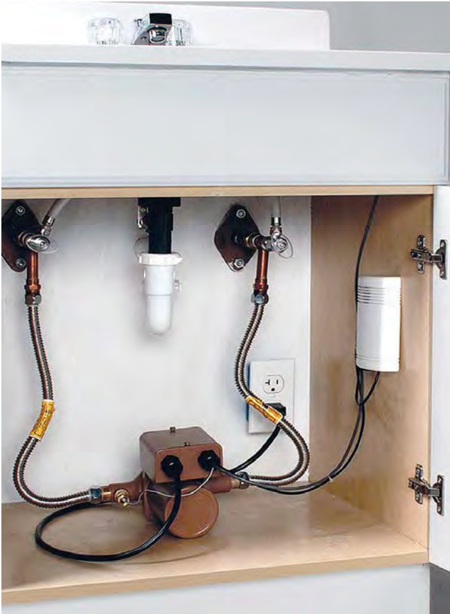
An on-demand recirculation system (with small pump and control housed in a bathroom or kitchen sink cabinet) saves water, but not energy for water heating.
