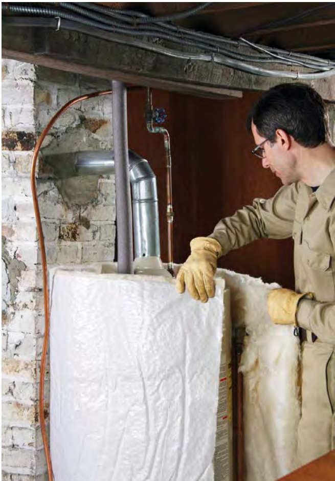
While many water heaters have significant insulation, wrapping one with an insulating water heater blanket can save even more energy.
