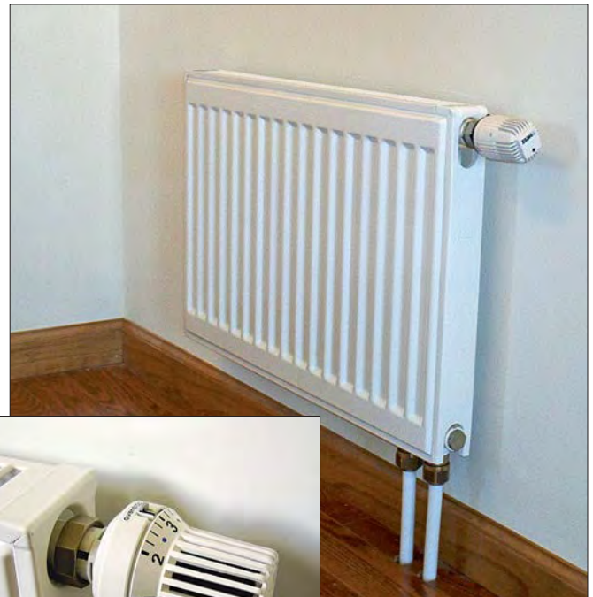
A panel radiator with an integrated thermostatic radiator valve.
