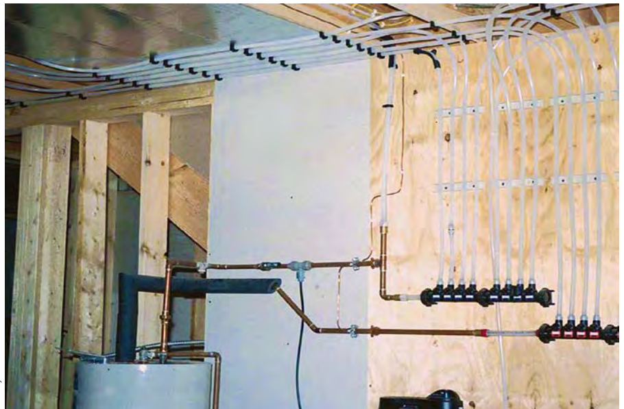
This “home-run” plumbing system routes individual lines to their own fixture or appliance, reducing friction losses from elbows and fittings.
