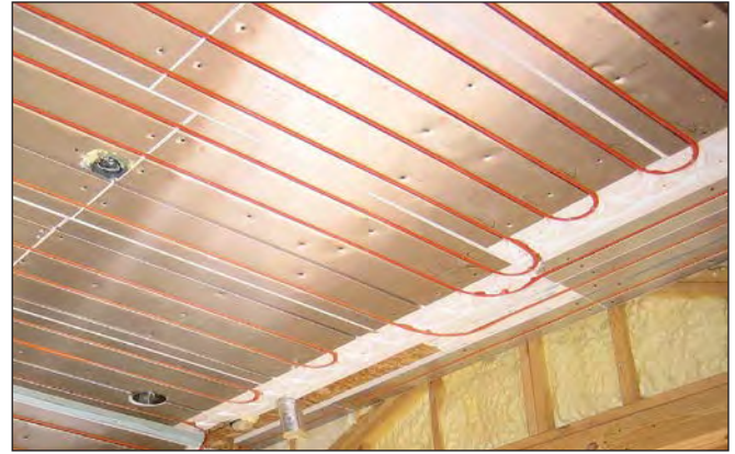
A radiant ceiling system is installed in much the same way as a radiant wall system.
