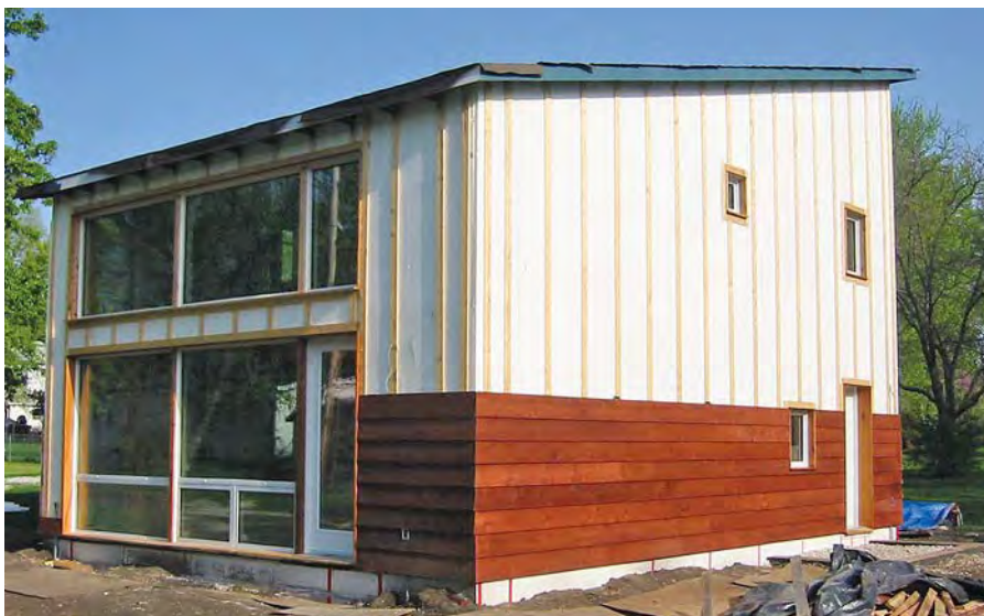
Klingenberg's I-joist solution, before and after wrapping with rigid foam insulation. Furring strips screwed to the I-joist flanges through the foam provided a vented rain screen and a place to attach the siding.
