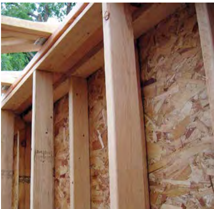
Two approaches to double-stud walls: Separated by a gap that will be filled with insulation, both staggered studs (right) and aligned studs (left) help minimize thermal bridging.
