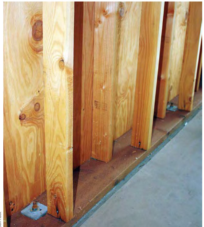
Two approaches to double-stud walls: Separated by a gap that will be filled with insulation, both staggered studs (right) and aligned studs (left) help minimize thermal bridging.
