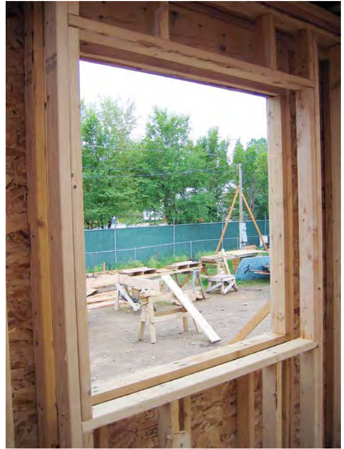
Door and window framing in a double-stud wall is more complex compared to standard framing.
