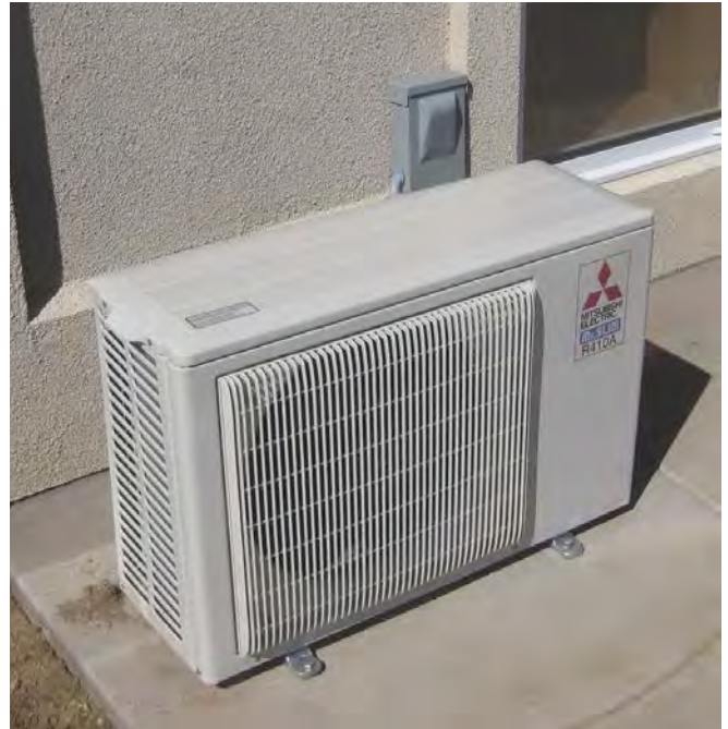
The minisplit exterior unit dumps the heat pulled out of the interior. In winter, the unit can run in reverse to produce heat.
