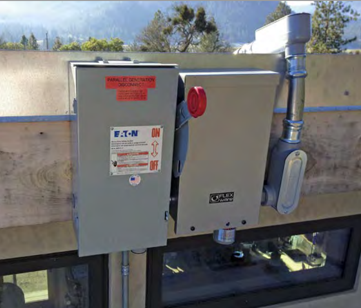
The DC disconnect (left) and the combiner, with its six fuses (right), are mounted on the north roof's fascia.
