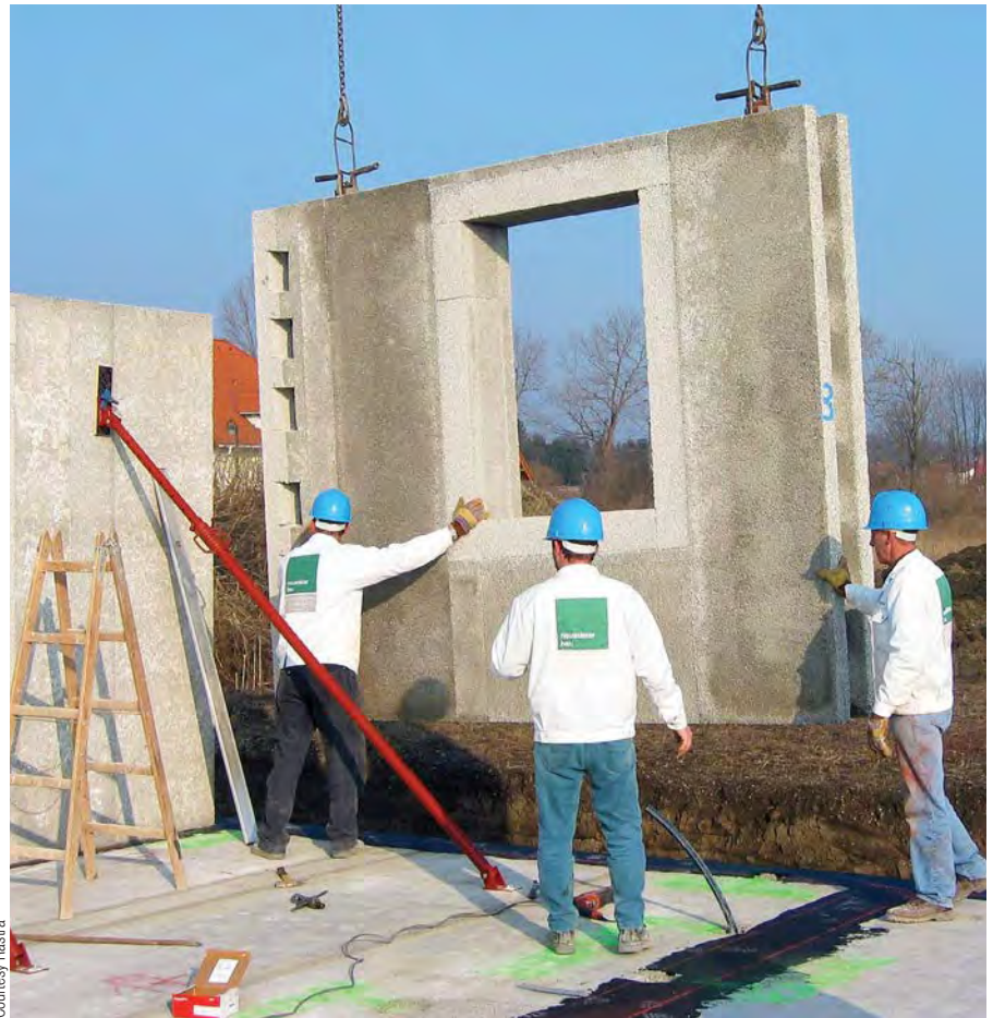
Larger Rastra ICF panels require heavy equipment to lift.
