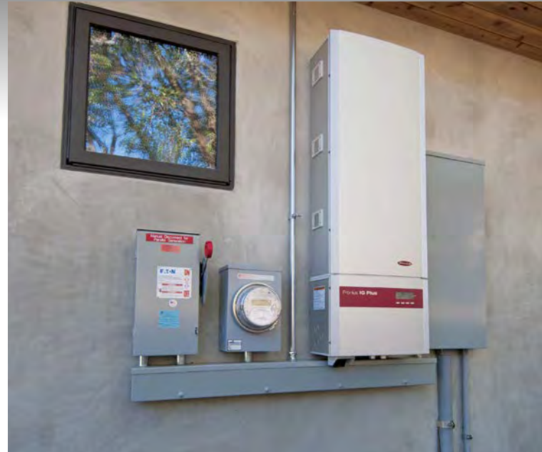
The power wall on the north side of the house with (L to R): AC disconnect, production meter, inverter, and household mains panel.
