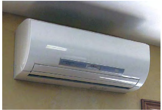
Small and fairly unobtrusive minisplit indoor units require no ducts.
