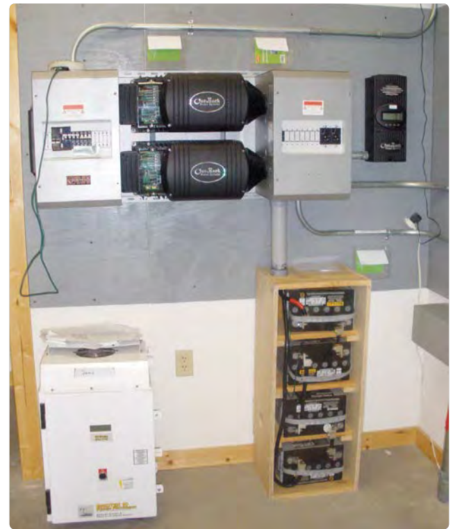
The RE systems' balance of system (BOS) components, including the charge controller, battery bank, inverters, and DC and AC load power centers.
