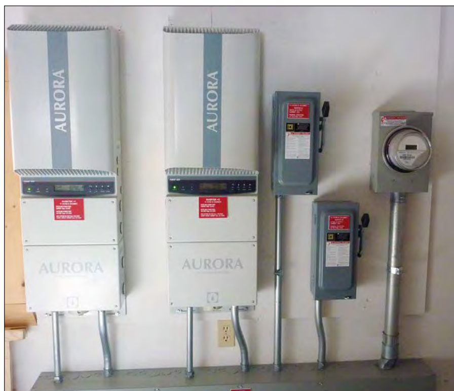
The Metzlers' 10 kW system uses two transformerless string inverters as well as typical balance of system equipment, including AC disconnects and a PV production meter.
