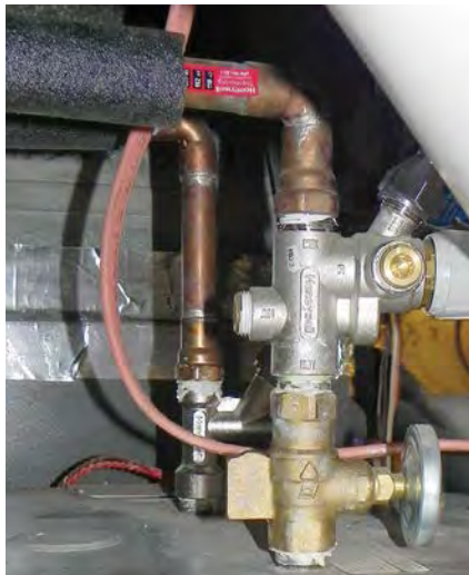
A side view of the top of the tank showing the thermometer that measures the tank's output temperature (the nearest copper pipe riser). Above it is the Honeywell adjustable mixing valve. The pink electrical cable is the 240 VAC electricity for backup water heating. The two twisted pair wires in the background connect to unused sensors (for active, not passive, systems) in the Bradford White tank.
