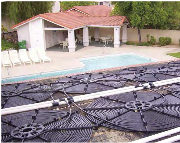
Unglazed coil-type collectors are best plumbed in parallel to reduce friction and preserve their solar collection efficiency.
