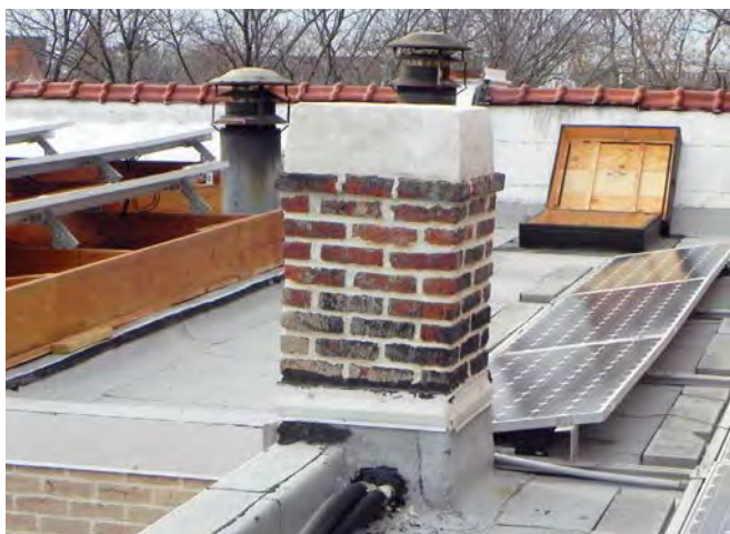
The chimney was removed and capped at roof level so it would not shade the PV modules.
