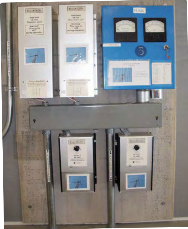
Diversion controller, dump loads, and DC panel.
