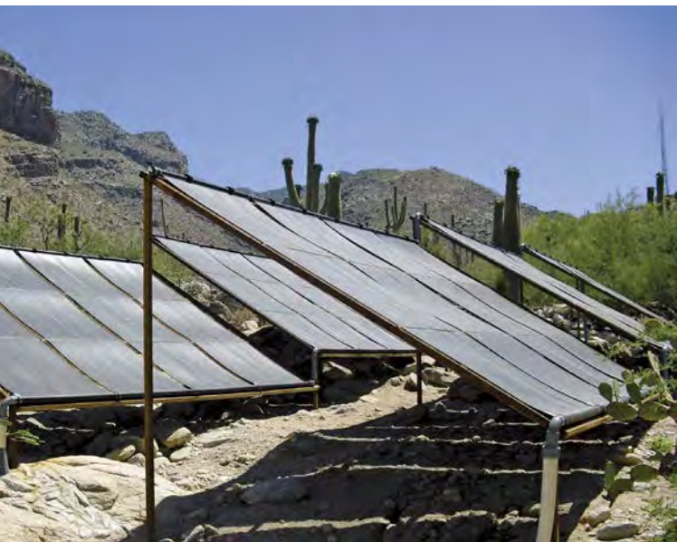
Flexible unglazed flat-plate collectors require a support framework if they are mounted at an angle, and tie-downs for wind protection.
