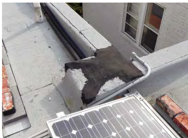
The old flue is now the chase for the foam-insulated PEX tubing going to and from the SHW collector.
