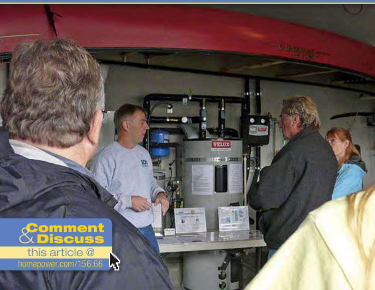
Mike Davis of SOS Plumbing explains the Clarks' Velux solar water heating system.
