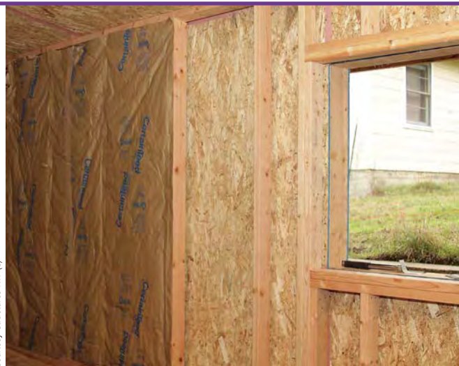
A nonloadbearing 2-by-4 wall inside the SIP wall provides room for additional insulation.
