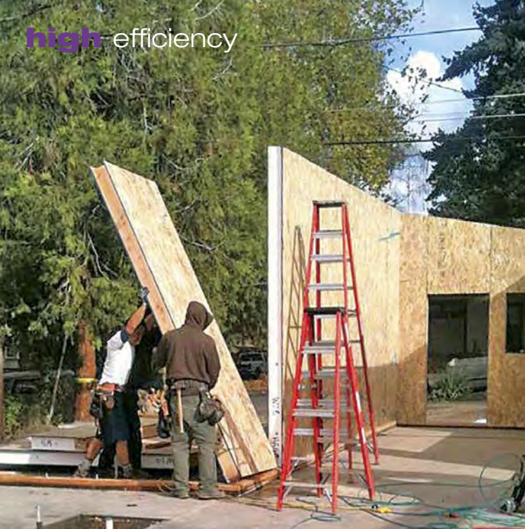
Custom-cut structural insulated panels go up fast, and insulate well with little air leakage or thermal bridging.
