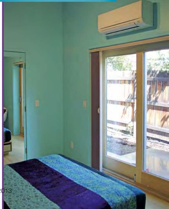
Right: The wall-mounted minisplit air handler in the guest bedroom is unobtrusive.
