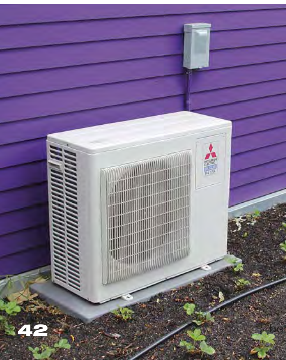
A minisplit heat pump that helps heat and cool the home with minimal energy input.
