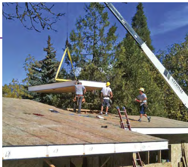
The 12-inch-thick SIP roof is placed by crane.
