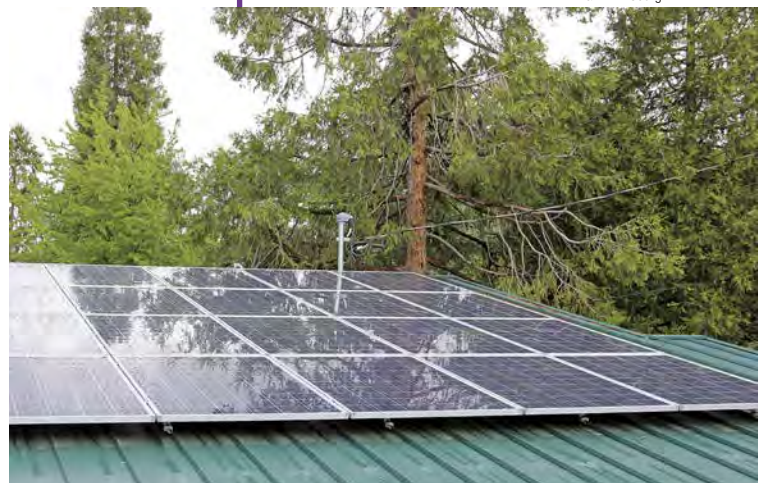
Part of the 12 kW PV array.
