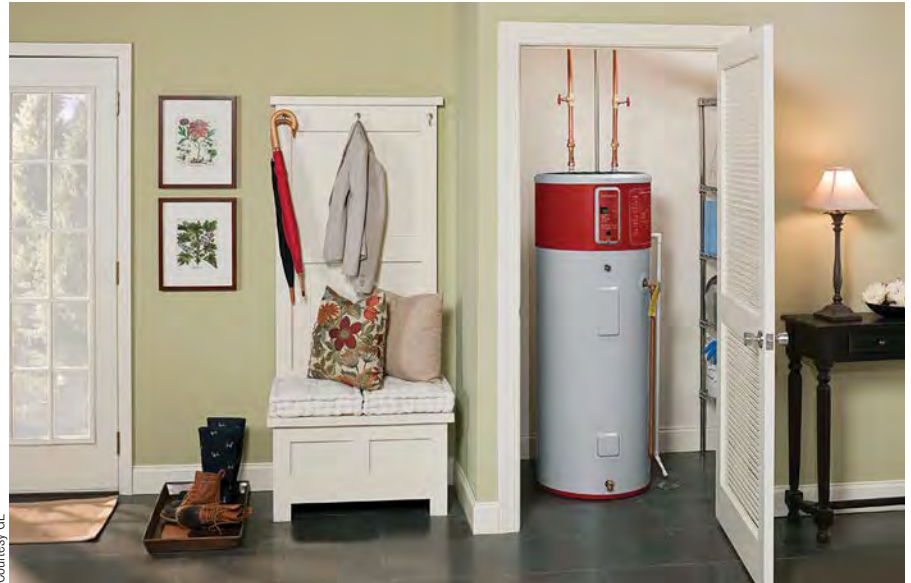
Heat-pump water heaters may have a slightly different footprint than conventional water heaters. Since they draw heat from the surrounding air, it is important to consider their location. With its louvered door, this closet essentially shares the same airspace with the living room.
