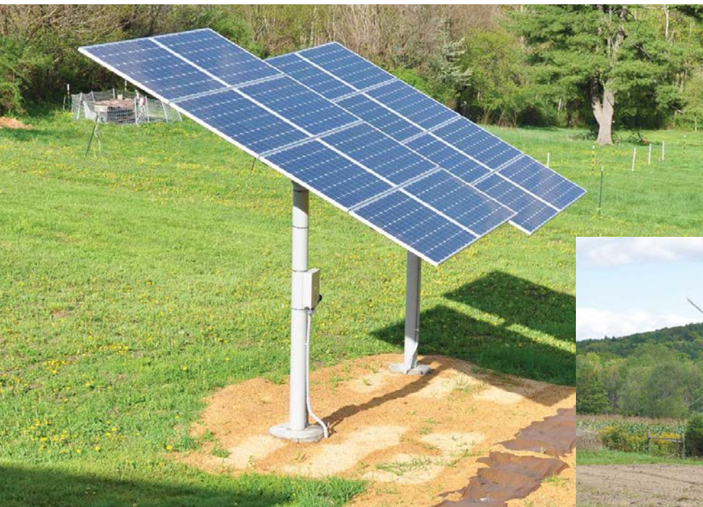
Much of the 21-foot lengths of the mounting poles are encased in concrete to handle the wind loads on the large arrays.
