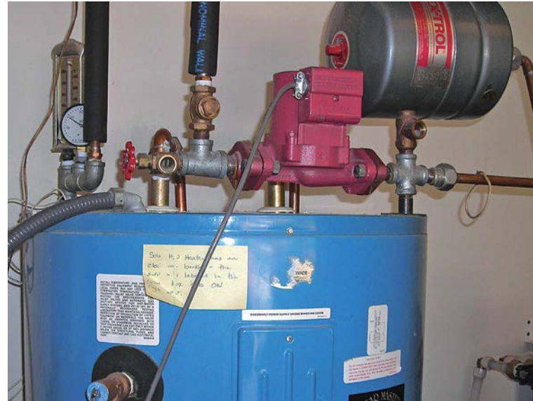
A vertically oriented pump shaft (shown above) will increase wear and tear on the bearings. Pumps should always be mounted with the motor axis horizontal.
