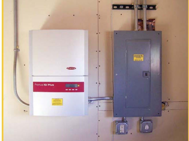
A single inverter (left) supplies a distribution panel (right) tied to the utility grid and to household loads.
