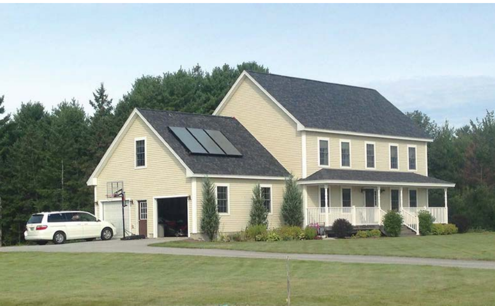
Flush-mounted collectors blend aesthetically with the roof and have less wind-loading, but are dependent on having a favorable roof pitch.
