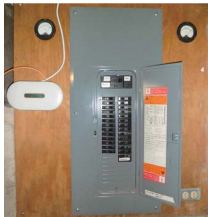
The Enphase Envoy production meter, which lives near the service panel, communicates to the Enlighten Web interface.
