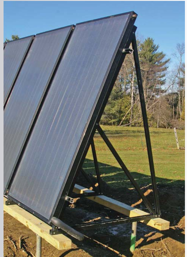
Foundations for ground-mounted systems must be installed below the frost line in areas subjected to freezing soil.
