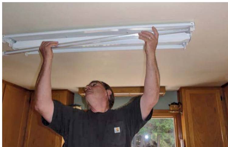
Step 5: Reassemble wiring cover and install LED bulbs.
