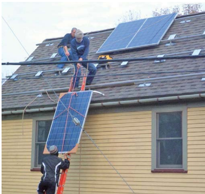
Homeowner and volunteer labor helped reduce installation costs. After rebates and projected production incentives, the calculated cost was about $1.16 per installed watt.
