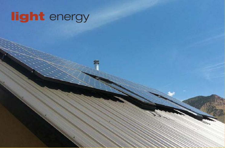
The 2.94 kW grid-tied PV array provides all of the home's electrical energy needs.
