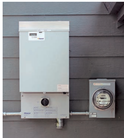
Above: A PV Powered 2,500-watt inverter, production meter, and disconnect (not shown) round out the balance-of-system components for this grid-tied installation.
