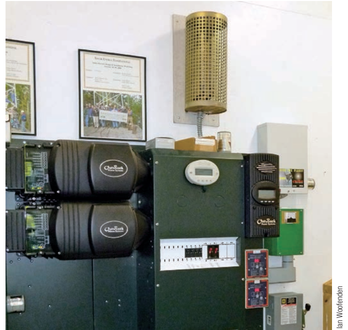
An air-resistance heater diversion load (inside a protective cage) is mounted above the power-conditioning components of a wind/PV system.
