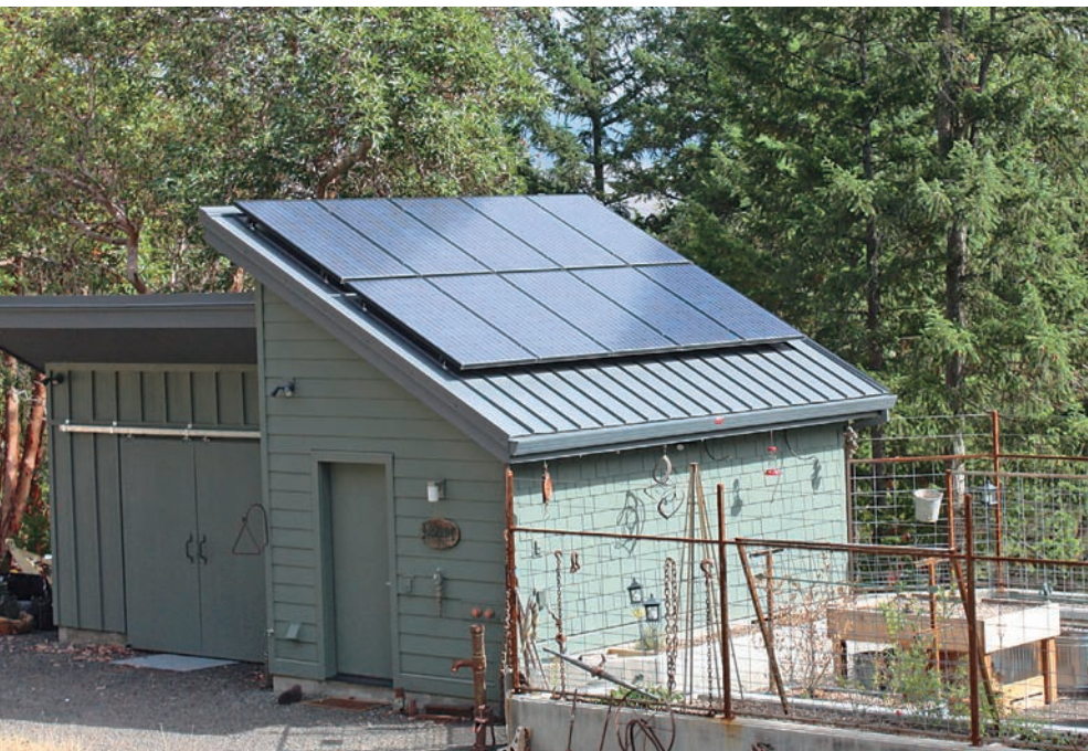
Ten 235-watt Sharp PV modules on the roof of the garden shed provide 65% of the Ashers' energy needs.
