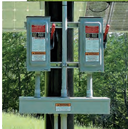
Above: To comply with NEC requirements for ungrounded PV systems, a two-pole disconnect was installed for each of the two source circuits.
