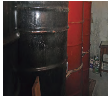
Eighteen tons of water act as thermal mass to store and moderate heat.
