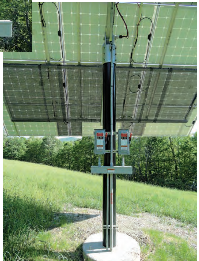
Right: The DP&W top-of-pole, adjustable-tilt mount sits on 8-inch schedule-80 steel pipe. Note the covering protecting the wiring where it is at a reachable height.
