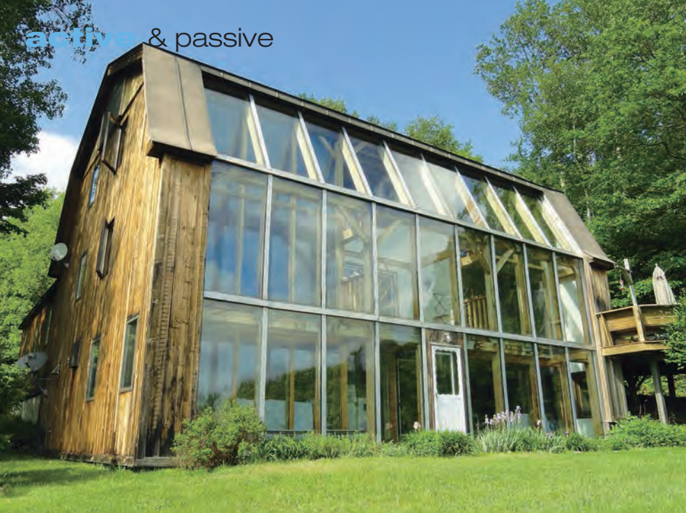
The glass south wall is separated from the living area by a full-height greenhouse that collects the solar-heated air.
