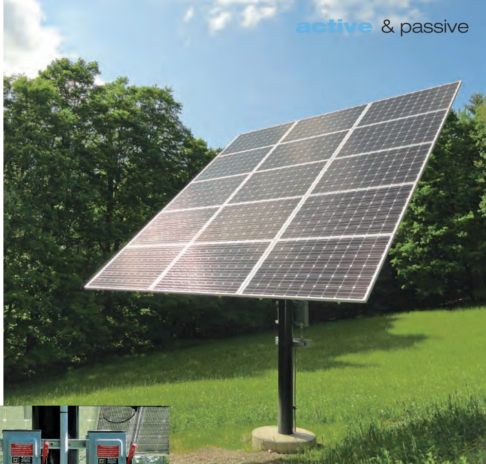
Fifteen SolarWorld PV modules totaling 4.2 kW.
