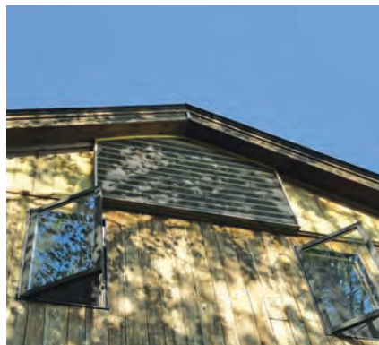
Excess heat is mechanically exhausted through gable-end vents.
