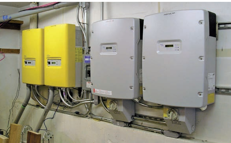
This classic AC-coupled system consists of 10 kW in the two gray SMA America Sunny Boy inverters; 8 kW in the Sunny Island inverters (yellow); and 10 kW of sealed AGM batteries (not shown) for storage.
