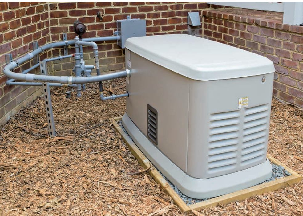
Left: A larger generator may be a permanently installed unit, with natural gas or propane fuel piped to it. Autostart is an option, but won't activate online fast enough to keep computers up.
