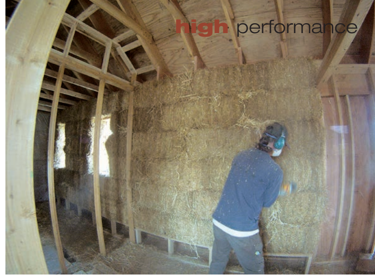
Straw-bale walls help improve thermal performance naturally.
