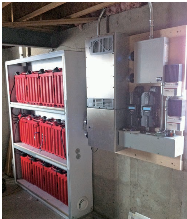
Below: This combo DC- and AC-coupled system has 5.4 kW that are DC-coupled through an OutBack Radian inverter; 6 kW are channeled through an AC-coupled inverter (not shown). MidNite charge controllers serve the DC-coupled system, while Morningstar controllers operate a diversion load for the AC-coupled system (protecting batteries from overcharge). Surrette flooded lead-acid batteries provide about 34 kWh of energy storage.
