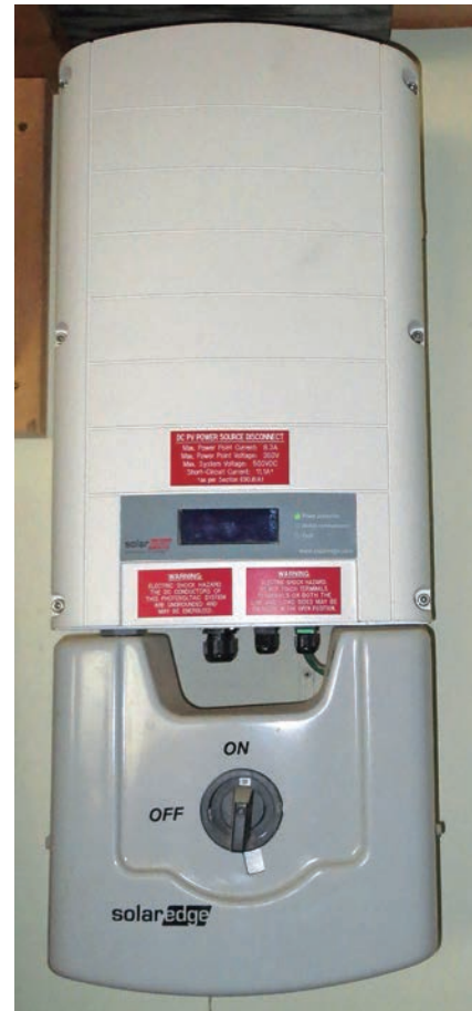
A SolarEdge 5 kW batteryless grid-tied inverter allows for another 1.25 kW of future expansion.
