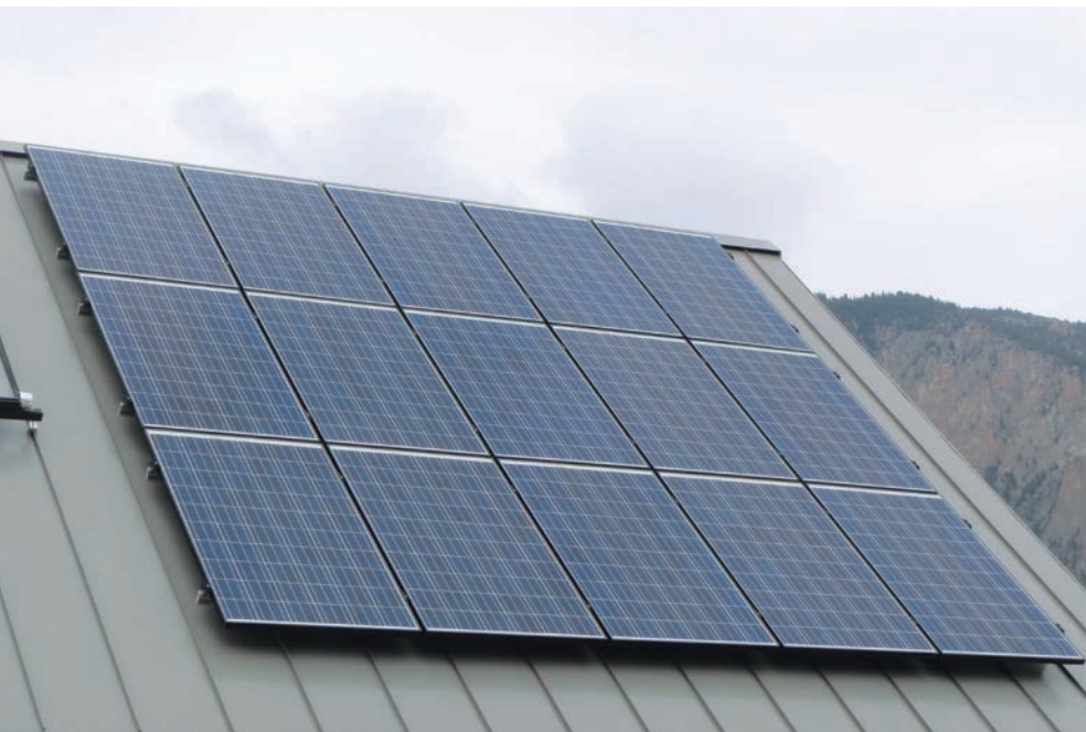
Fifteen REC Solar 250-watt PV modules provide about 5.88 megawatt-hours of energy per year.
