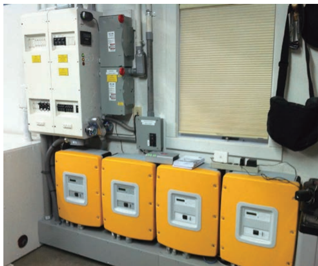
This large AC-coupled battery backup system includes 26 kW of PV power connected to five Sunny Boy inverters (not shown) and four Sunny Island inverters (shown below).
