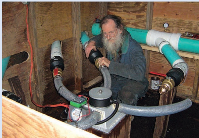
Smooth sweeps reduce friction losses in this four-nozzle turbine manifold.
