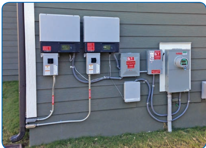
Poorly routed and sloppy arcs of LFMC affect the aesthetics of this BOS area.
