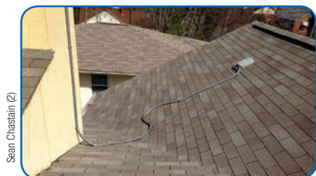
Left: Please don't. This is a recipe for trapped ice and debris, and stress on the conduit and wire.
