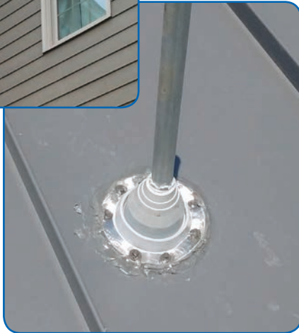
Right: A flashed and caulked boot roof penetration can transition into the attic or through to the eaves when a vaulted ceiling is present.
