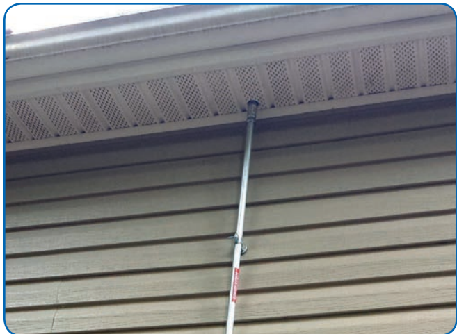
Through the soffit, or directly down and through the roof, is a good way to get out of the attic.
