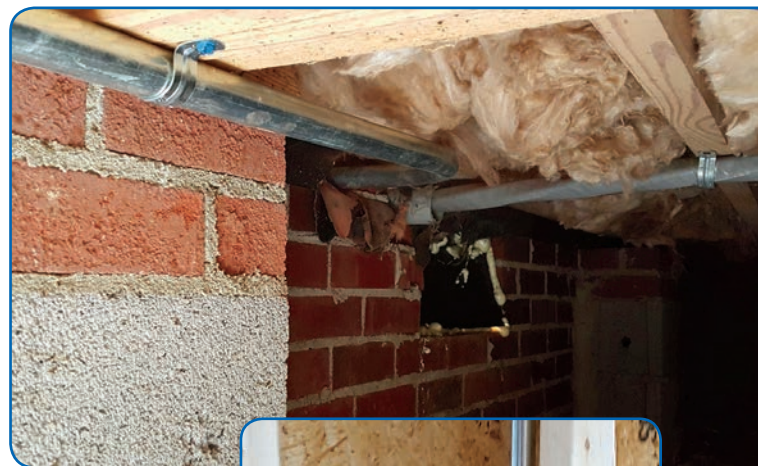
Above: Conduit routed through a crawlspace, following the joists.
