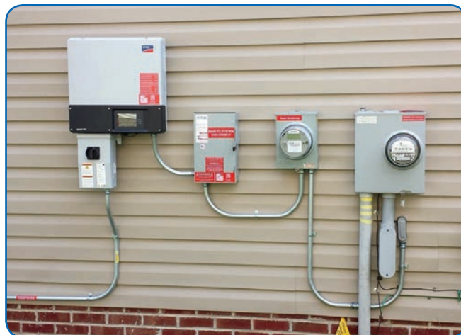
The inverter and BOS are the perfect place for clean conduit work. Here, strategic component placement and clean sweeps make the installation look professional.
