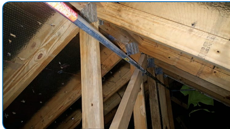
Above: Well-routed EMT follows the rafter layout and is 10 inches below the roof deck.
