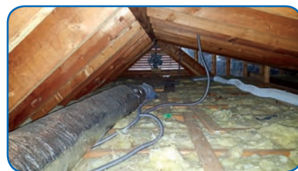
Right: Poorly installed FMC wanders through the attic.
