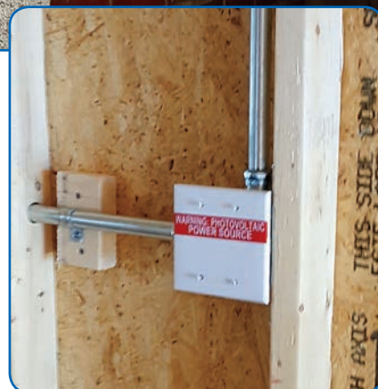
Right: Junction boxes must not be hidden in walls; this exterior cover will show after the drywall is finished.
