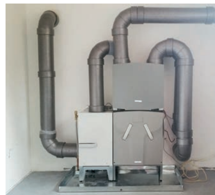
The Zehnder ventilation system, from left to right: ComfoFond L Eco 550 ground-loop-based preheater; ComfoAir 550 energy recovery ventilation unit; and ComfoCool 550 cooling unit.
