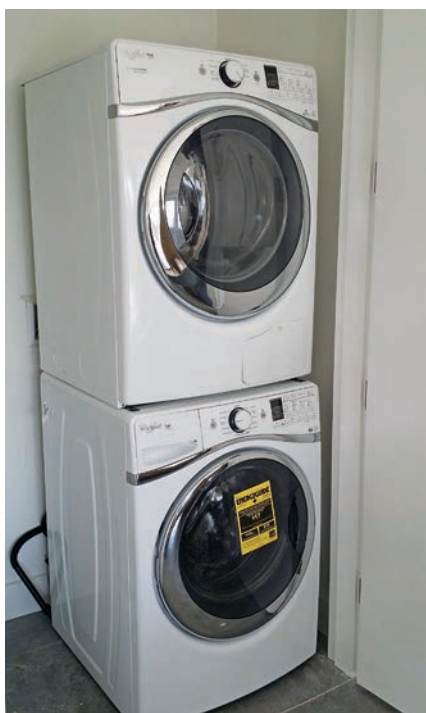
The Whirlpool Hybrid Care dryer, which has a heat pump, doesn't require an external vent.
