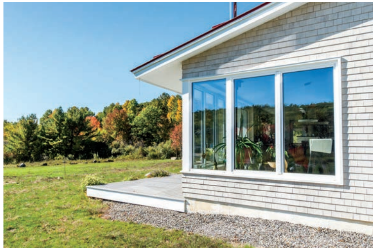
The large east windows gain morning light for quick warm-ups on winter days, while the west side is shaded, and protected from afternoon overheating.
