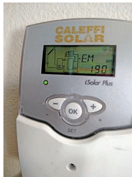
The solar thermal differential controller's high-temperature setpoint was lowered from 205°F to 190°F to prevent vaporization at the 7,000-foot elevation.
