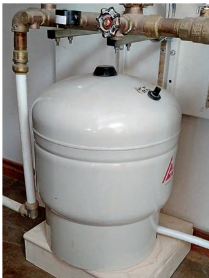
The substantial temperature difference between the 40°F incoming well water and 120 gallons of 170°F stored solar-heated water required replacing the original 4.4-gallon pressure tank with a 10.3-gallon unit.
