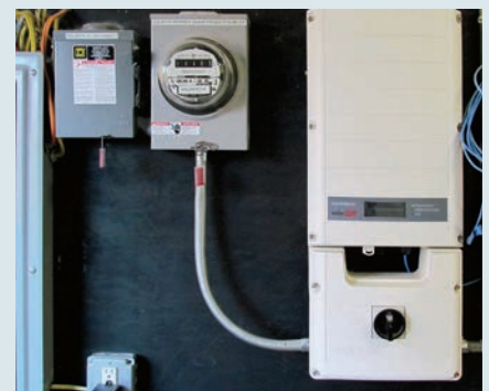
Right: The 7.6 kW SolarEdge StorEdge inverter.
