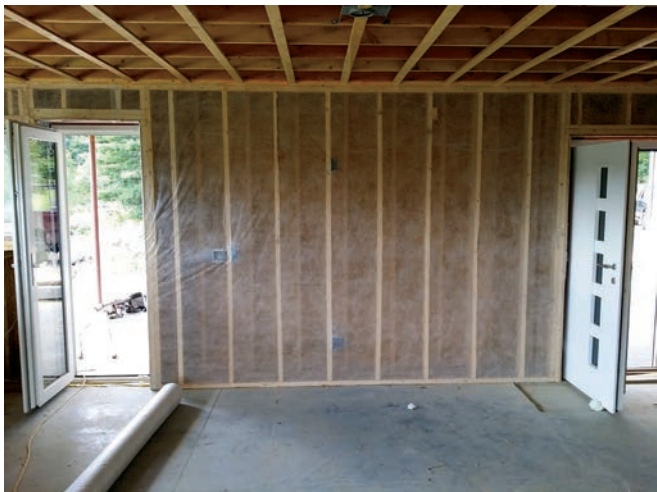
Twelve-inch-thick, double-stud walls were filled with cellulose for an insulation value of R-45. Ceilings are insulated to R-70; the floor is insulated to R-26.
