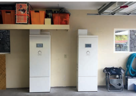
Two sonnenBatterie units provide 24-hour self-consumption of PV-generated energy without exporting to the utility.
