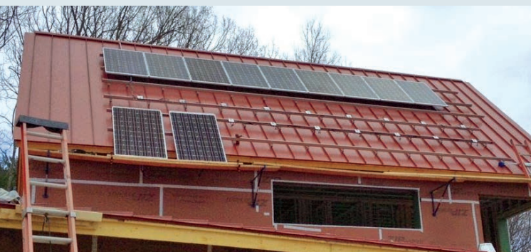
Left: The PV modules and DC optimizers during installation.
