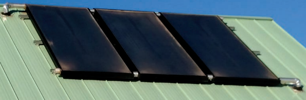
Three SunEarth 4-by-10-foot solar thermal collectors provide a substantial portion of domestic hot water needs, even during cold and cloudy periods.
