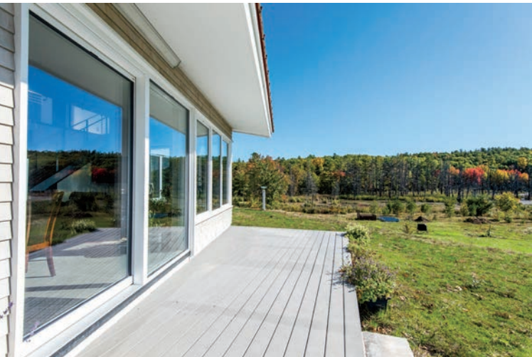
The main living area is angled slightly southeast from the main structure. Excess solar gain is controlled seasonally by large eaves.
