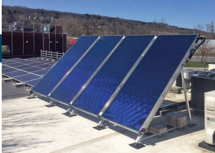
Solar thermal flat-plate collectors (above) and balance-of-system components (below) make up this SunMaxx solar water heating system.
