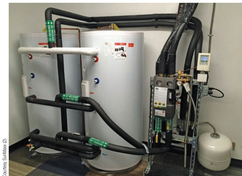
Solar thermal flat-plate collectors (above) and balance-of-system components (below) make up this SunMaxx solar water heating system.
