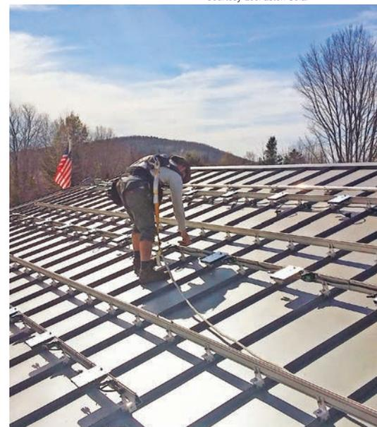
The advantage of standing-seam metal is that the standoff hardware attaches to the roof without any penetrations.
