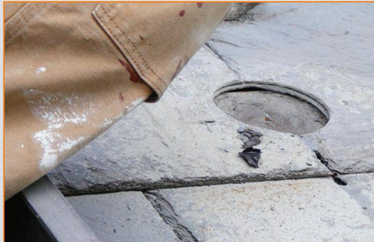
Slate tiles were drilled with a carbide hole saw.
