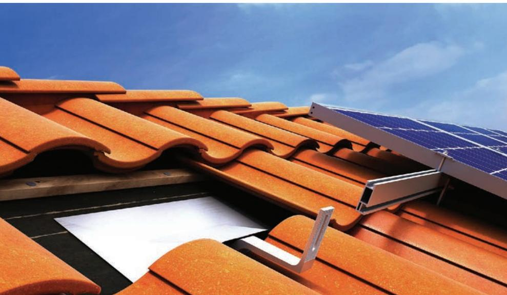
Left & below: Tile hooks like these by Quick Mount PV are designed to mount under a tile. The mount hooks between the courses of tiles.
