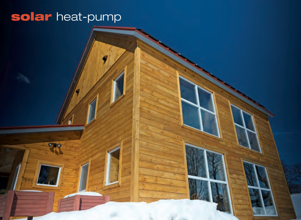
Above: The traditional post-and-beam frame was wrapped in structural insulated panels, giving the walls an insulative value of approximately R-40.
