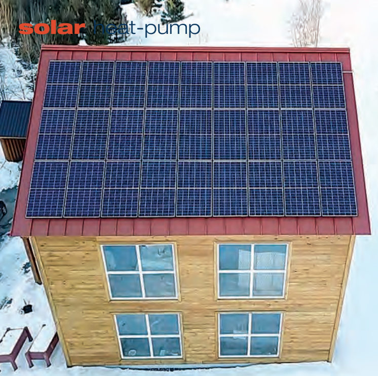
Left: The 7.83 kW PV array.
