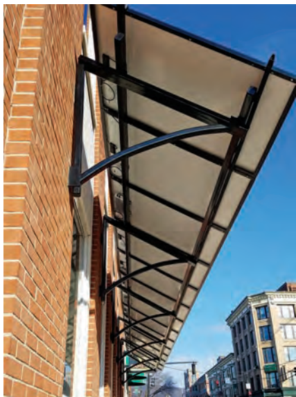
Left: The custom PV awning serves two functions: providing shade for the lower windows and generating energy.
