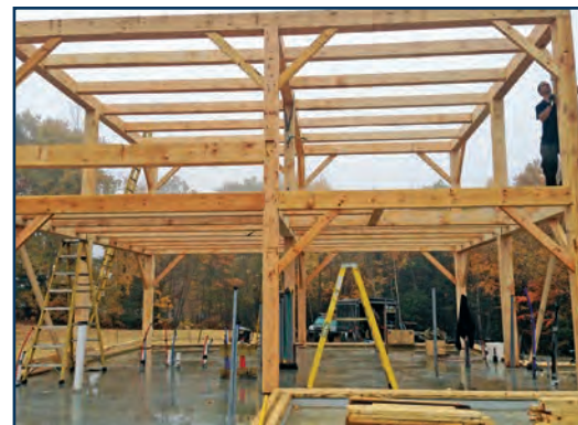
Above: The traditional post-and-beam frame was wrapped in structural insulated panels, giving the walls an insulative value of approximately R-40.
