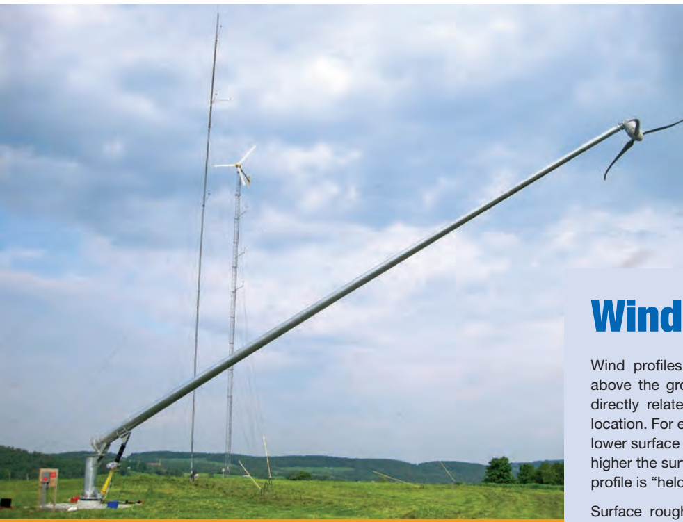
Left: A Xzeres Skystream, installed in 2013, produces nearly 1.7 MWh annually. Here, it is being tilted down for turbine maintenance.
