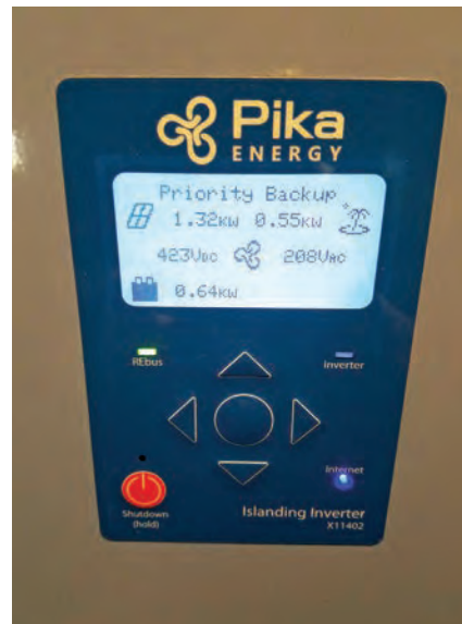
Right: The Pika Energy inverter display showing backup power being used during a grid outage.
