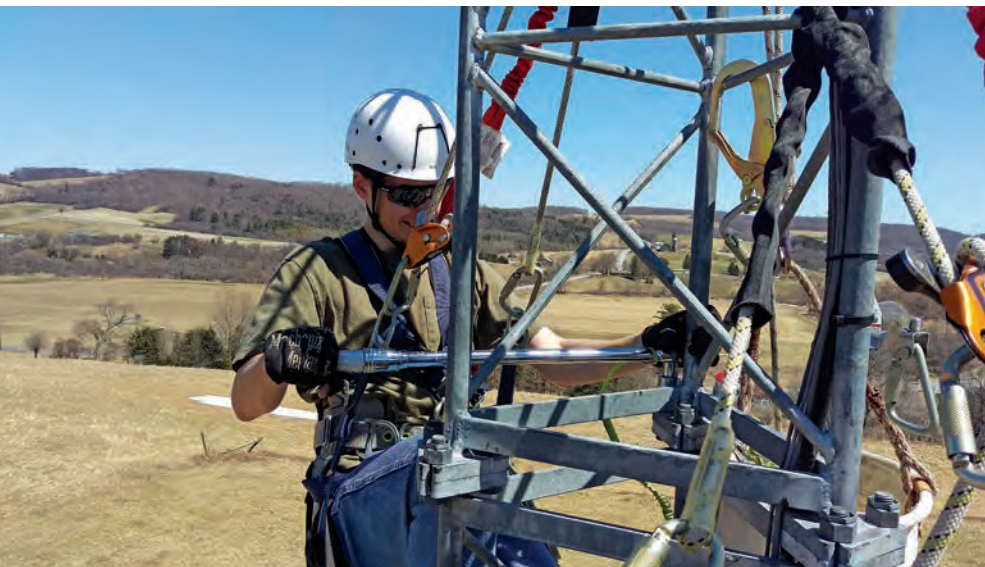
Above: Routine maintenance is more routine in this hands-on learning environment. Here, student Ben Wlock checks torque specs on the Bergey's 120-foot guyed lattice tower.
