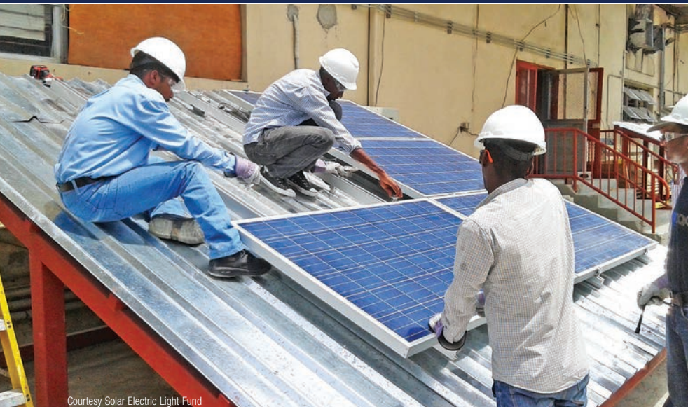
Haitian instructors install a lab-yard array during a “train-the-trainers” course.
