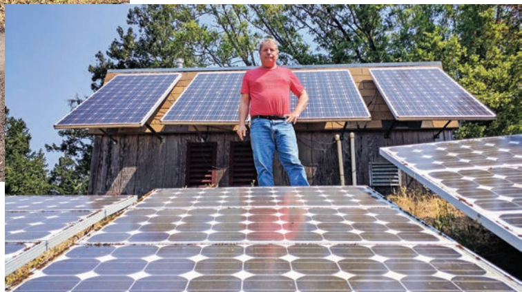
Mark Haynie, shown with several modules in the 4 kW PV array that provides electricity for his home and transportation.
