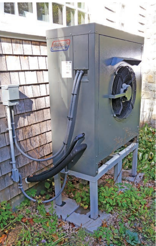
Left: The outdoor portion of a split-system heat pump by Nordic. The stand elevates the unit above snow level. Refrigerant tubing and electrical cables pass through the wall to the indoor unit.
