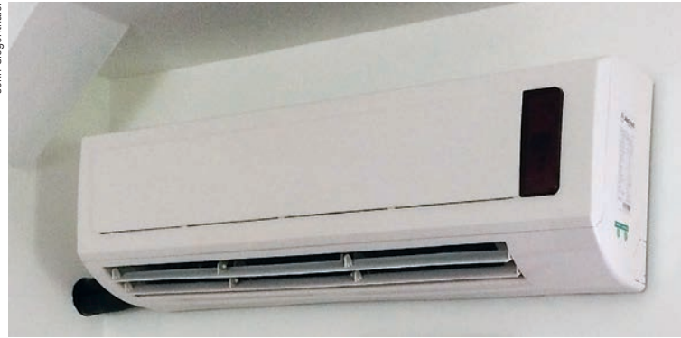
This wall-mounted air handler can be coupled to an A2W heat pump to provide space heating and cooling.
