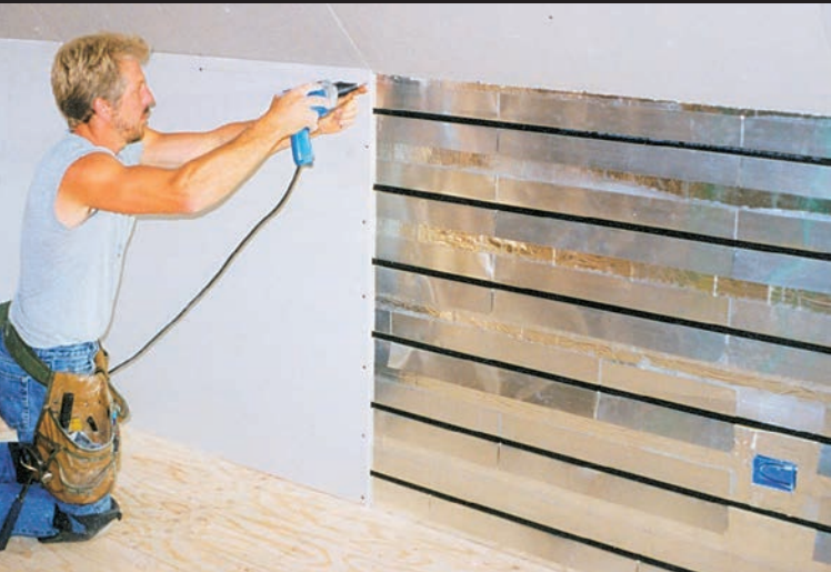
A radiant wall panel, also with PEX-AL-PEX on aluminum heat-transfer plates, installed behind drywall.
