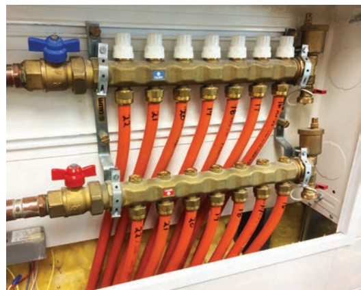
Below: A typical manifold station that supplies water to radiant floor-panel zones.
