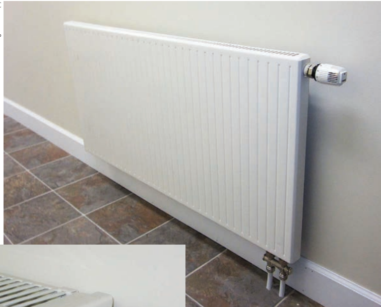
A typical wall-panel radiator with wireless thermostat. Although their origins are in Europe, panel radiators are now readily available in North America.
