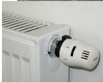
A typical wall-panel radiator with wireless thermostat. Although their origins are in Europe, panel radiators are now readily available in North America.
