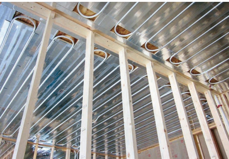
Radiant ceiling panels—1/2-inch PEX-AL-PEX tubing spaced 8 inches apart with aluminum heat transfer plates—prior to drywall installation.
