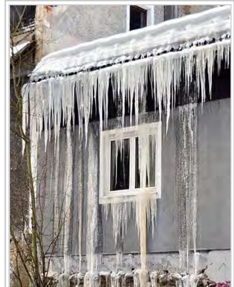
Icings resulting from water leaking through the roof due to an ice dam, caused by snowmelt on the roof.
