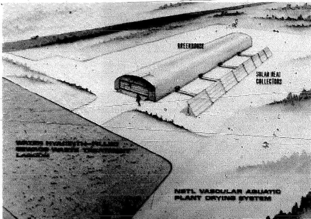
Solar energy is being harnessed to dry aquatic weeds in experiments at the National Space Technology Laboratories near Bay St. Louis, Mississippi. This system is connected to a process that farms water hyacinth on sewage effluent. (National Space Technology Laboratories)
