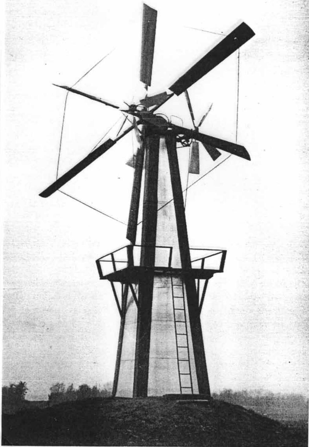
Modern re-construction of Type 0, for electrical power generation.
