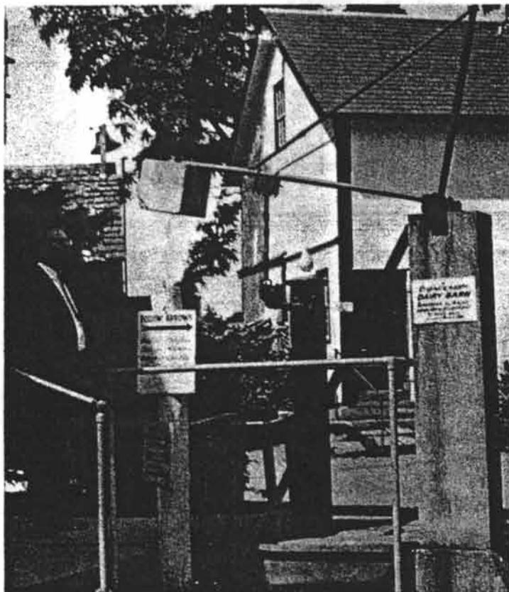
A reciprocating wire can transmit power from a water wheel to a point up to 0.8km (1/2 mile) away where it is usually used to pump well water. These devices have been used for many years by the Amish people of Pennsylvania. If they are properly installed, they give long, trouble-free service.
